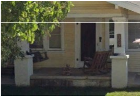
154 N Harwood Stucco masonry pilasters
