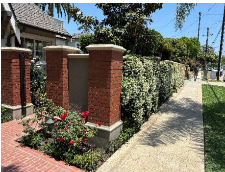
205 Pine St Solid wall with pilasters
