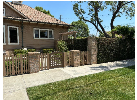
704 E Maple (kitty-corner) Brick pilasters and arbor
