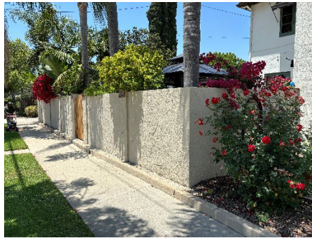
206 Pine St Solid wall with pilasters
