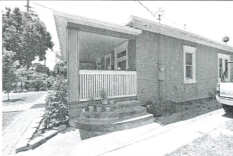
North elevation of porch and front of main house
