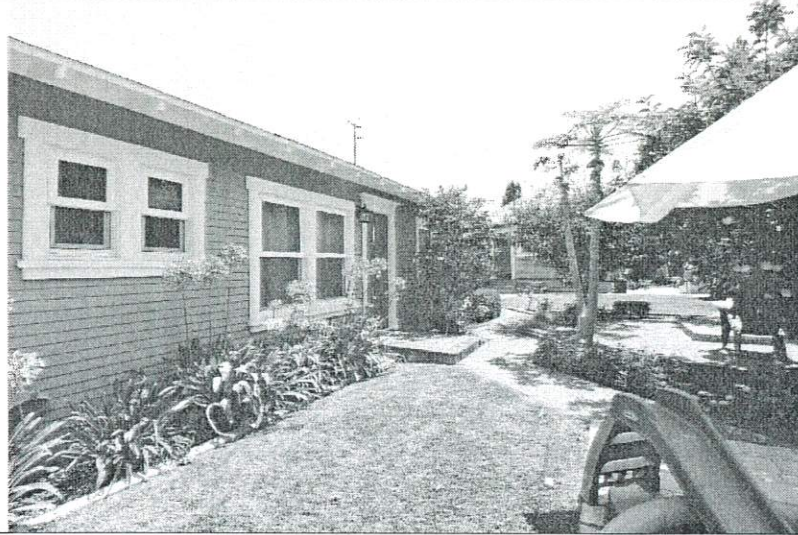
Carriage house facing northeast towards main house
