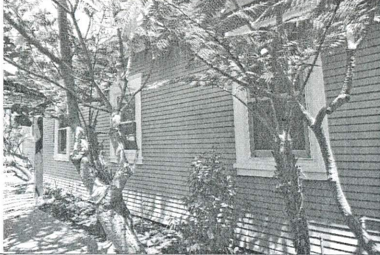
South elevation of main house (looking west)
