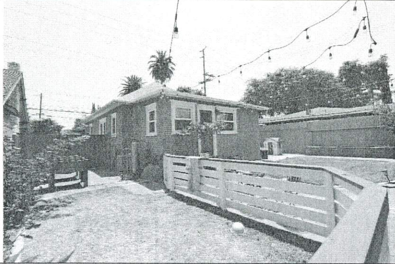
West elevation of main house (Northeast view)
