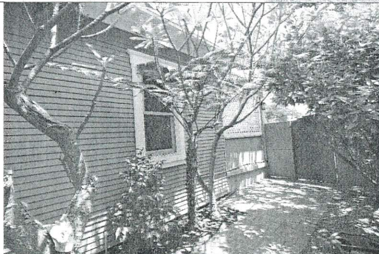
South elevation of main house (northeast corner)
