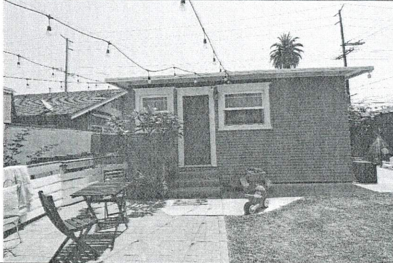
West elevation of main house
