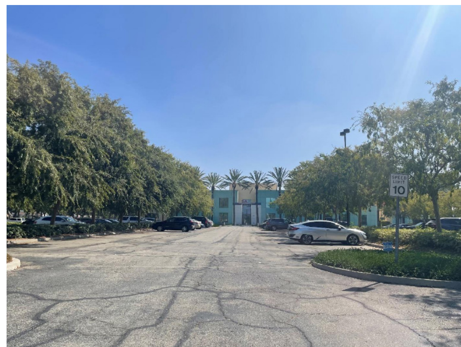
5 INTERIOR EAST SIDE OF SITE | LOOKING WEST
