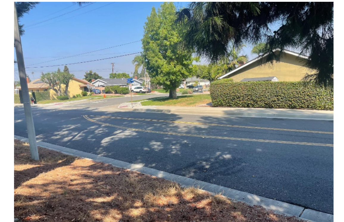
2 NORTHWEST ON FLETCHER AVE | LOOKING NORTH
