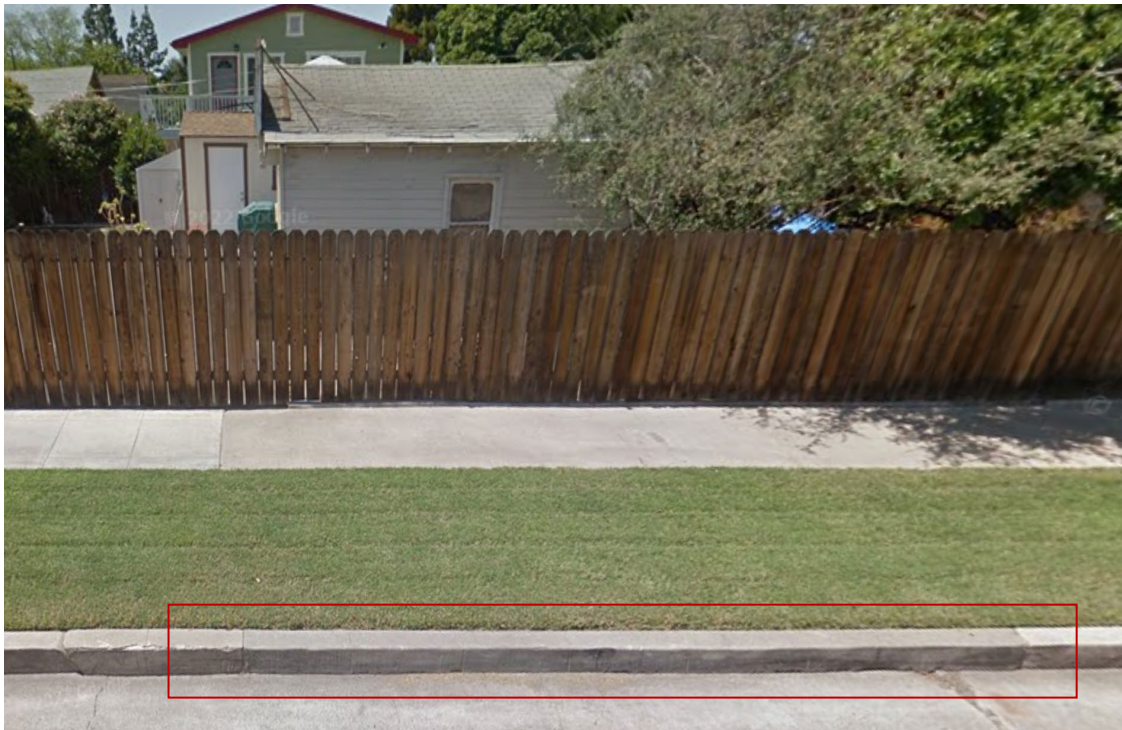
Section of Curb Infill at Previous Driveway
