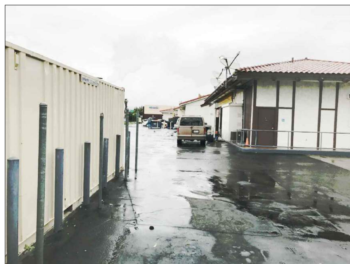
SIDE OF STATION NEXT TO CONTAINER
