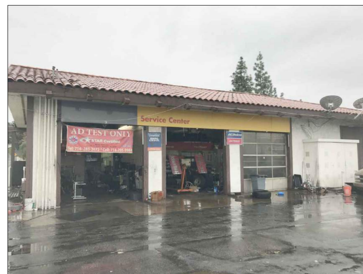
SERVICE STATION (REAR)
