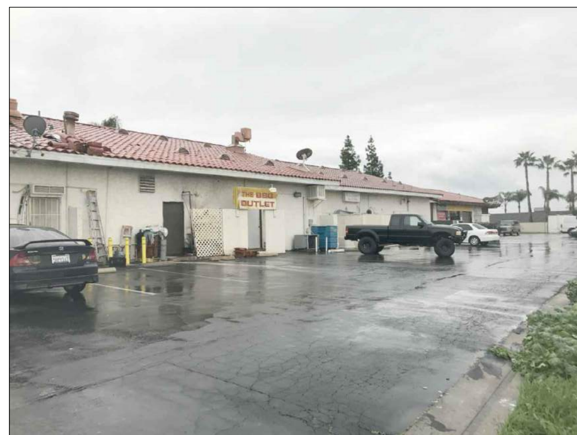
REAR OF RETAIL CENTER
