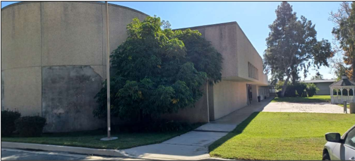
5-SOUTH ELEVATION FROM NORTH PARKING LOT
