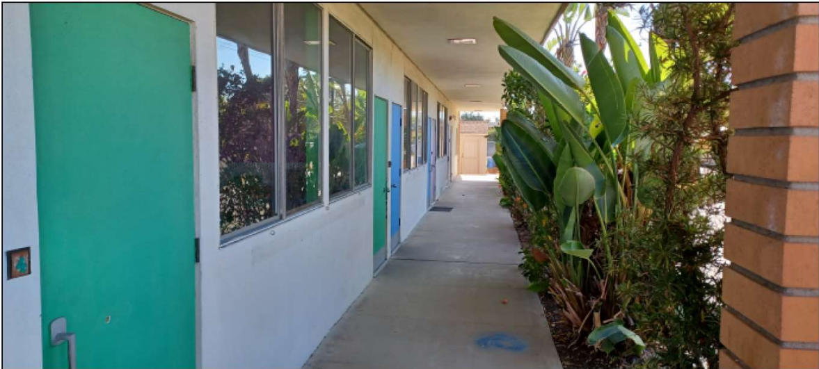
4—EAST ELEVATION FROM WEST DRIVEWAY
