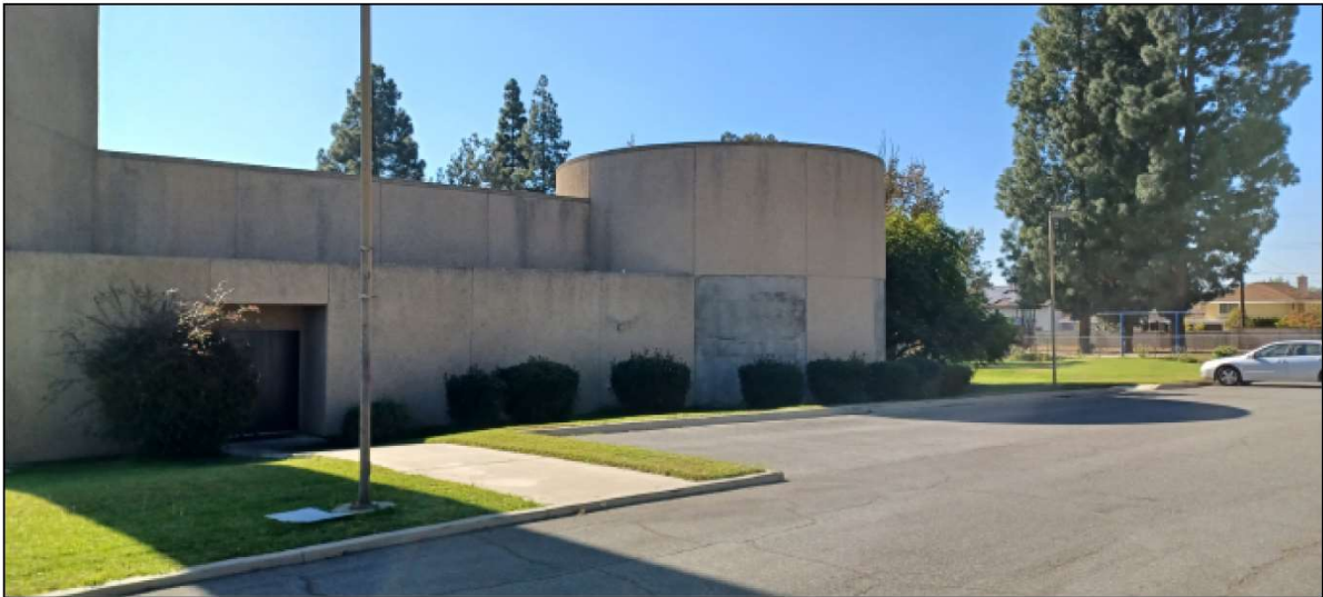
4—SOUTH ELEVATION FROM NORTH PARKING LOT
