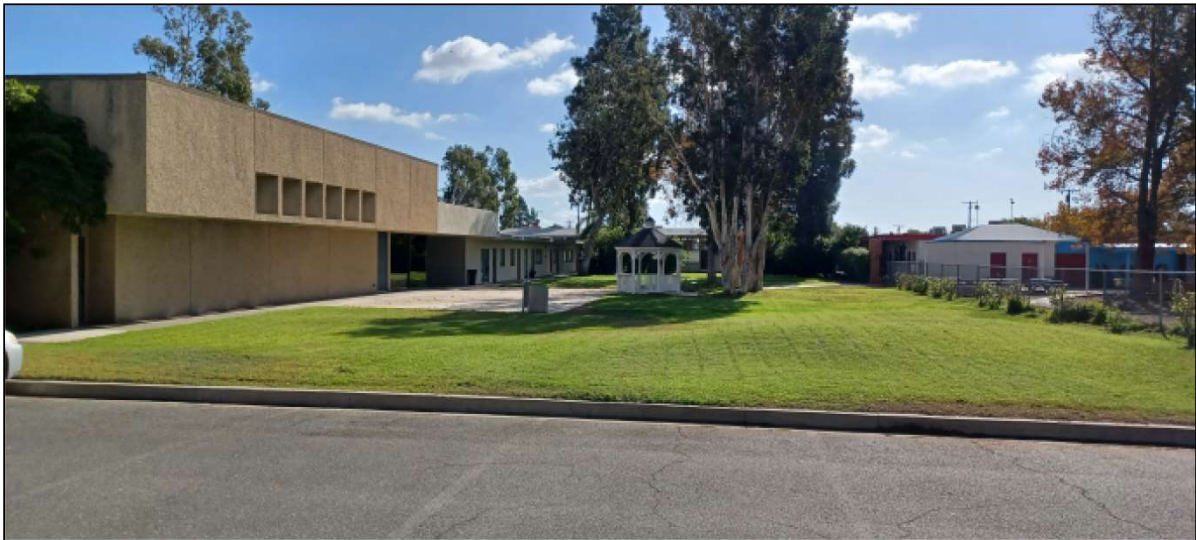
10—SOUTH ELEVATION FROM NORTH PARKING LOT
