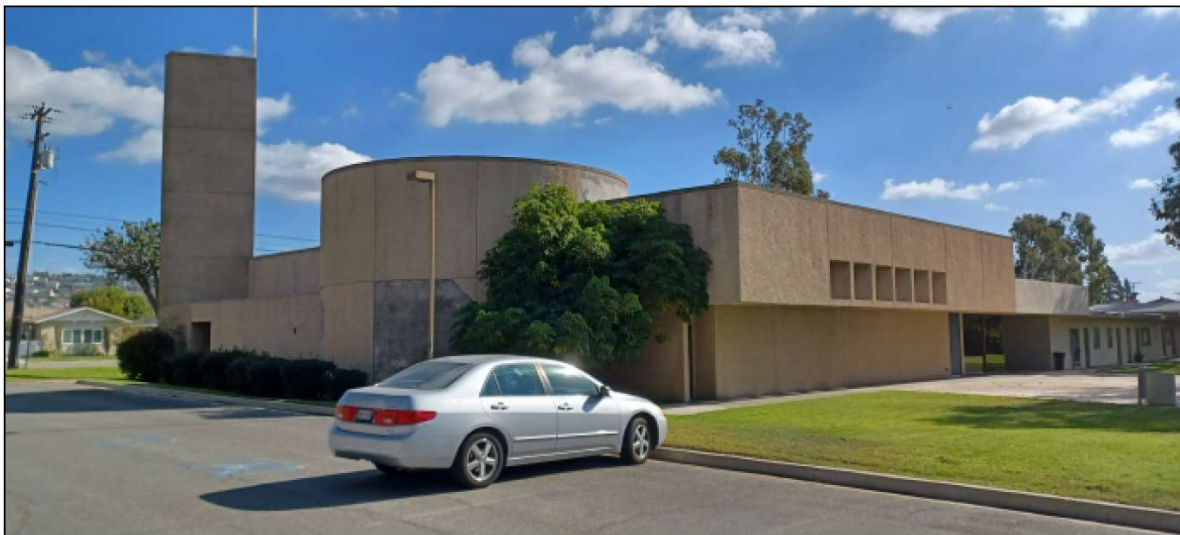
6-SOUTH ELEVATION FROM NORTH PARKING LOT
