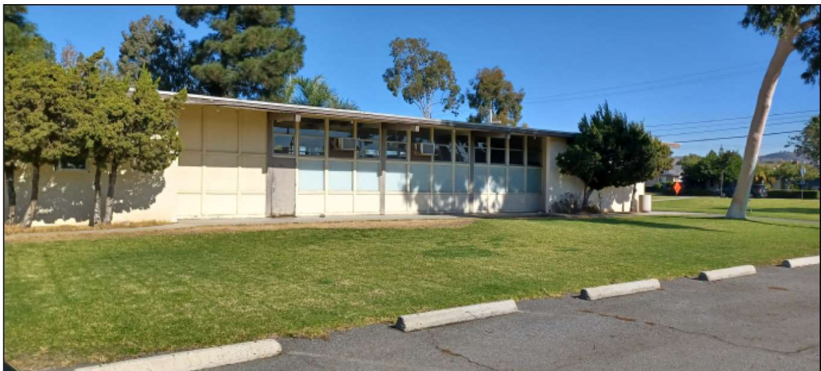
12—NORTH ELEVATION FROM SOUTH PARKING LOT
