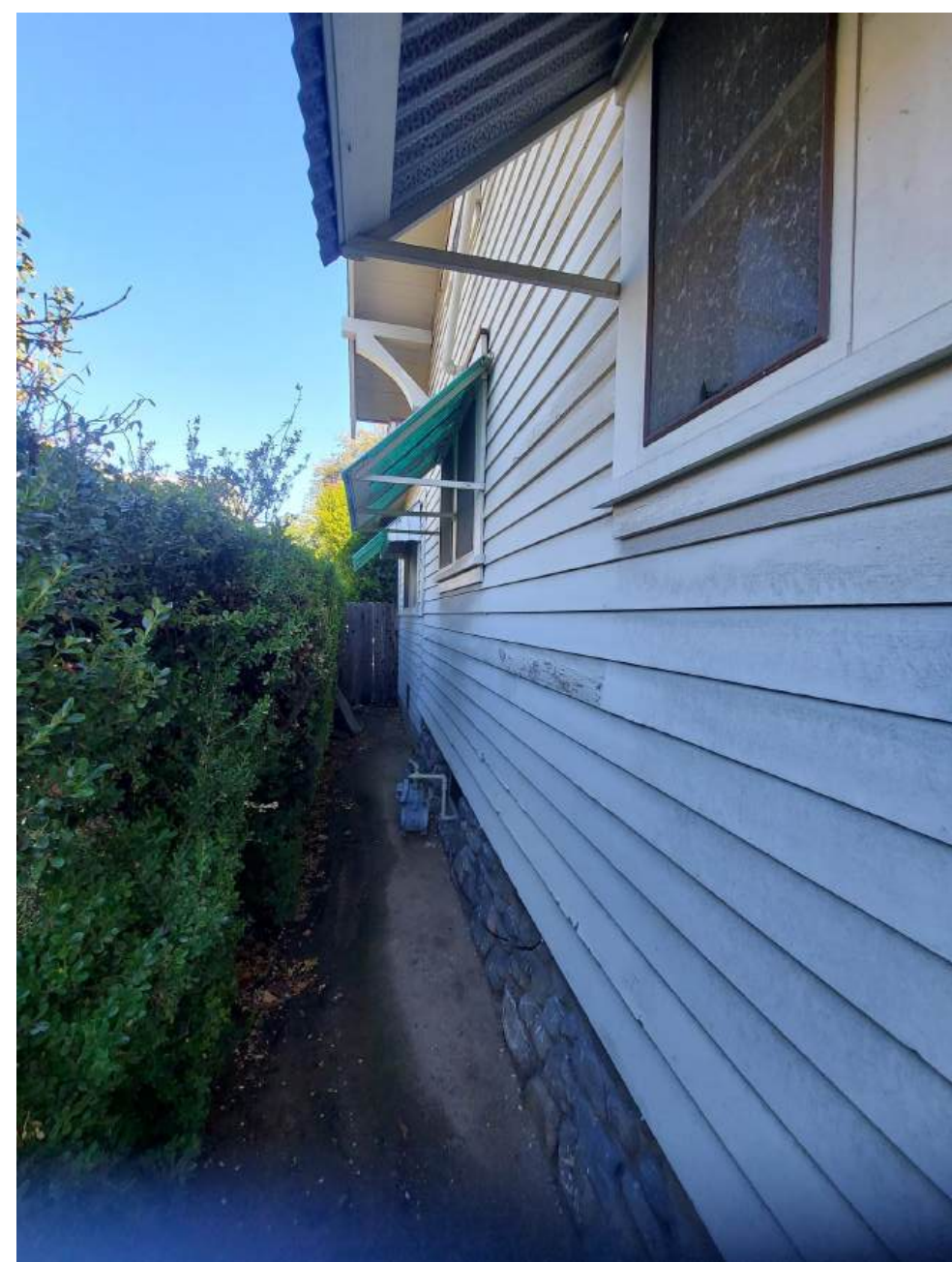
View of west facade from side yard
