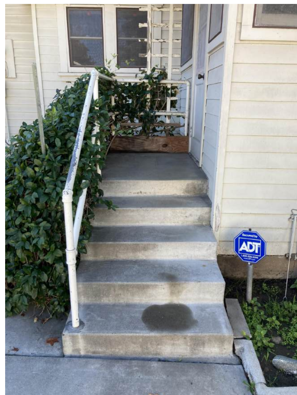
Closeup view of staircase being removed at addition
