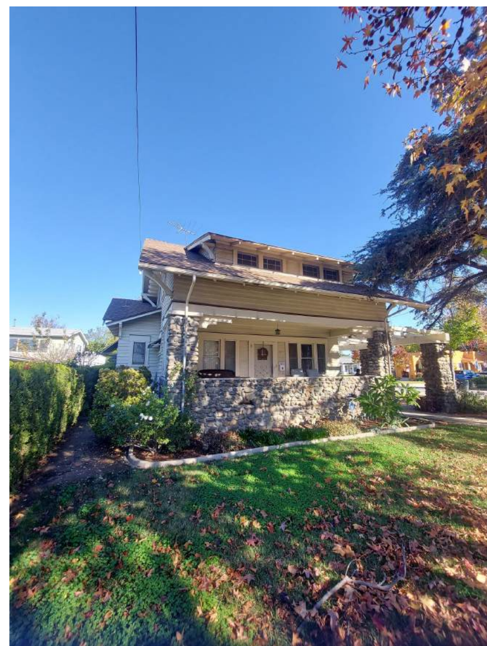
View of southwest corner of main residence from street
