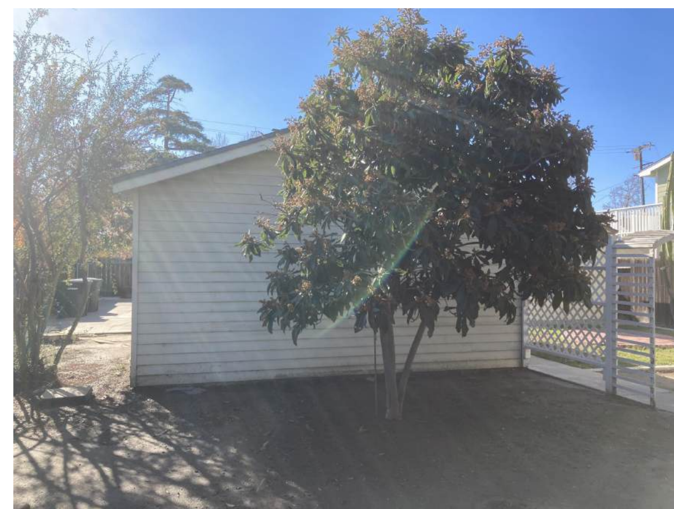
View of north facade of existing garage
