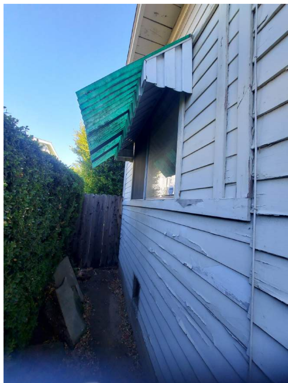
View of west facade looking at area of previous addition
