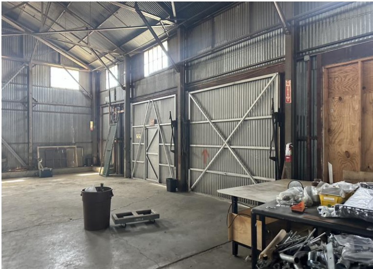
Figure # 4: Structural reconstruction of Hangar Building, southwest façade of interior wall surface interior cross bracing.
