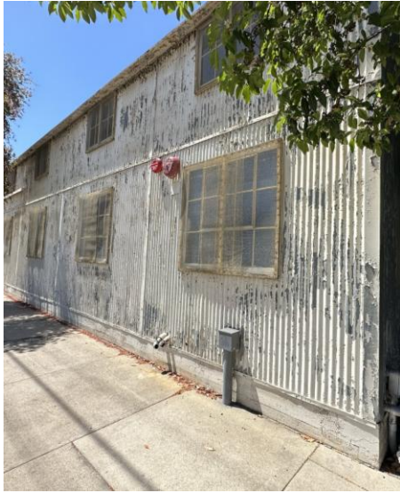
Figure # 28: primary south façade detail of corrugated metal panels and trim where repair and rehabilitation are required actions.
