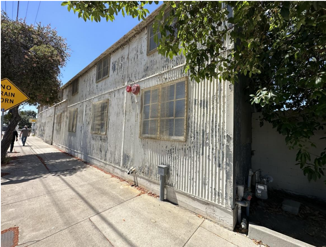
Figure # 9: primary south façade detail, oblique view to the west. Noted condition of corrugated metal wall panels above cast-in-place concrete curb walls. Noted deteriorated condition of wire mesh screening set in wooden frames and then applied to the face of the steel frame windows.
