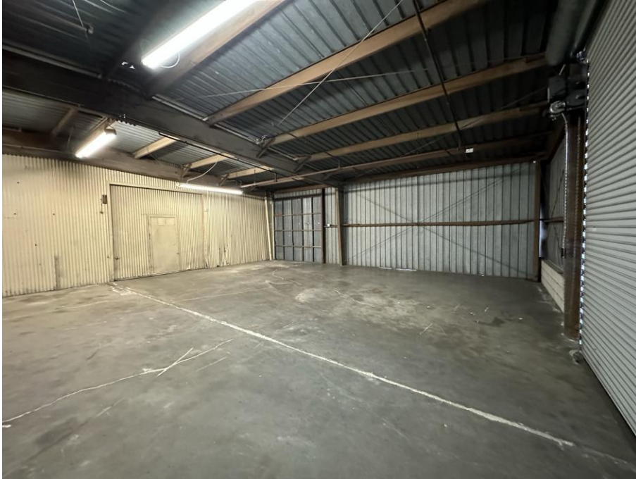
Figure # 12: north façade addition, view to south; ramped slope floor is proposed to be filled in. Rear wall at left is the original north façade of the Hangar Building corrugated metal panel façade. If the north addition were proposed to have this wall removed to accommodate new program use, these original corrugated panels could be retained for re-use elsewhere if necessary.
