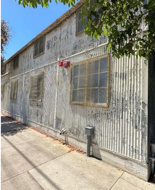
Figure #25: primary south façade detail, oblique view to west. Noted condition of corrugated metal wall panels above cast-in-place concrete pony walls. Noted condition of wire mesh screening set in wooden frames applied to face of the steel frame windows.
