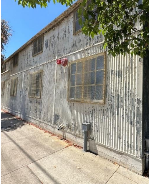
Figure # 27: primary south façade detail, oblique view to west. Noted condition of wire mesh screening set in wooden frames applied to face of the steel frame windows.
