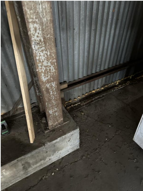
Figure # 15: Detail of the base of steel columns and a concrete curb at east façade interior wall. Noted that the curb terminates at the location of the original doorway opening in the east façade an atypical detail.
