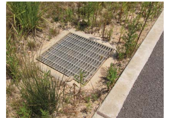
Appropriate drainage inlets for storm water overflow
