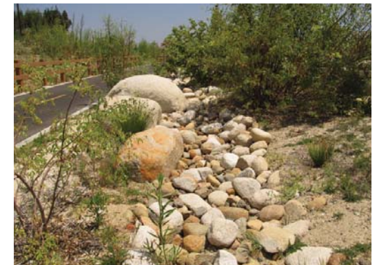
Cobble swales capture and filter water from storm events
