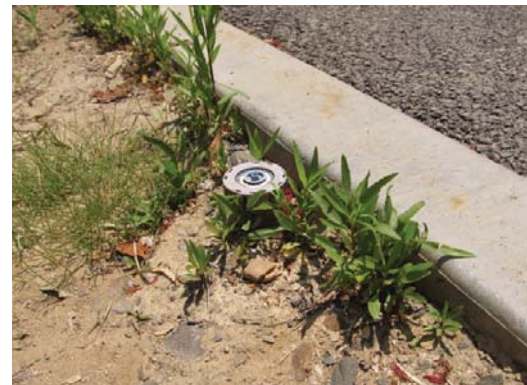
Reclaimed water irrigation system for planting areas
