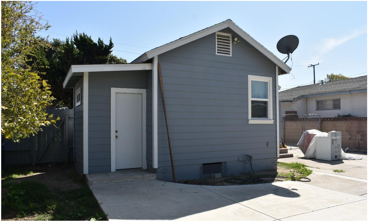
Image 7: Rear and secondary (north) façades, view southeast
