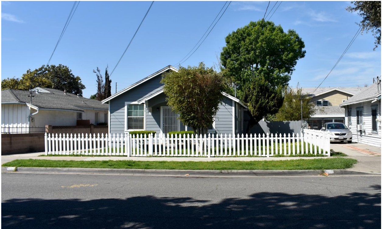
Image 1: Primary (South Parker Street, east) façade, view west
