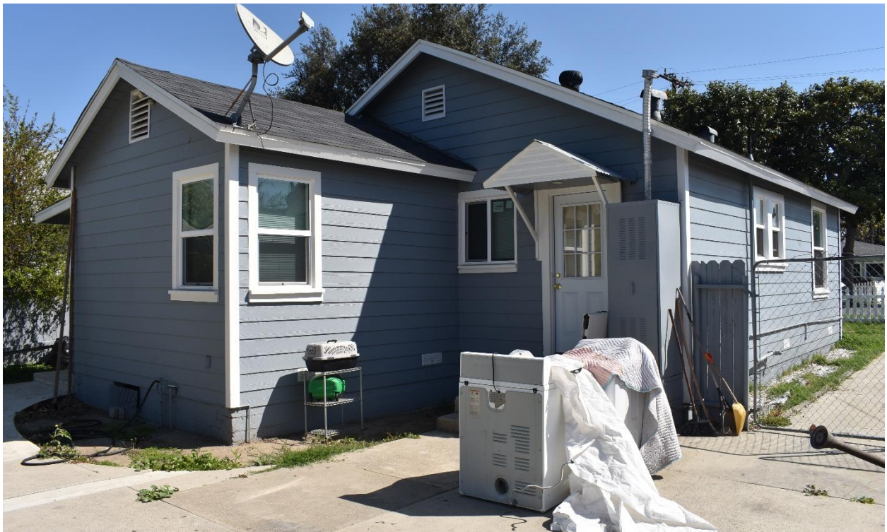
Image 6: Secondary (south) and rear façades, view facing northeast
