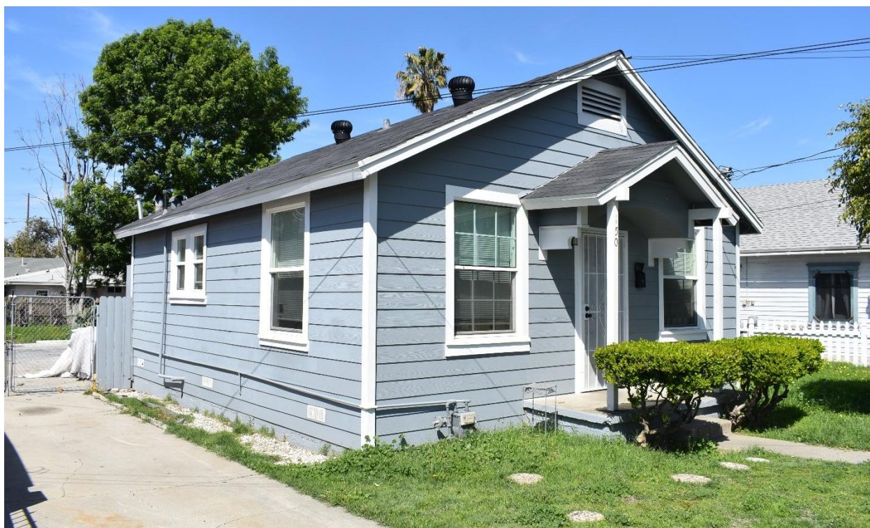
Image 3: Primary and secondary (south) façades, view northwest
