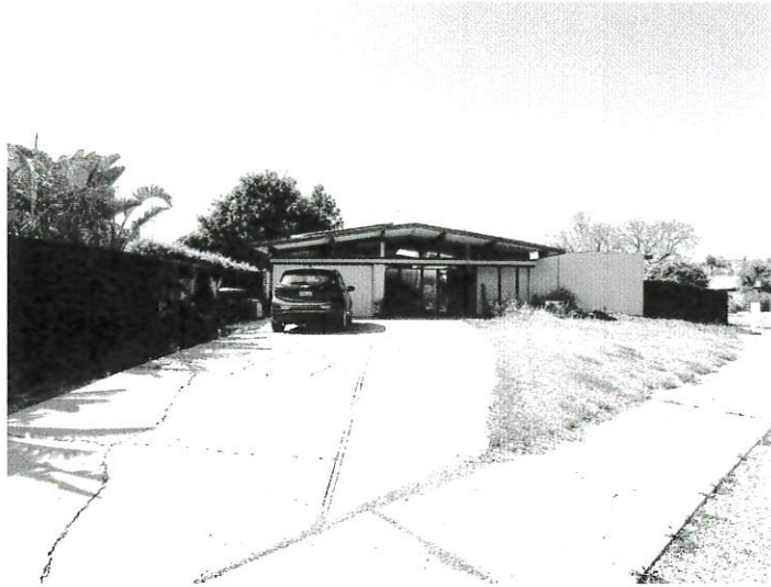
Image 01 South [front] Facade [Facing North] | May 9, 2024
