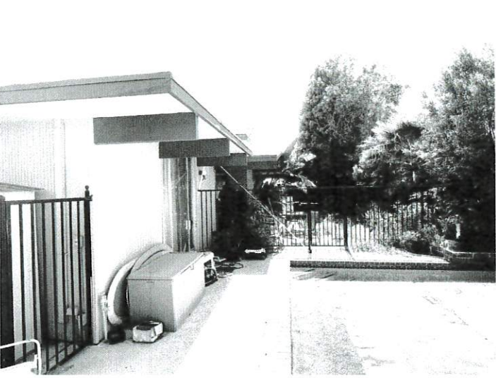
Image 05 North [rear] Facade [Facing West] | May 9, 2024
