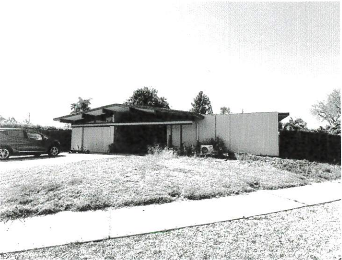
Image 02 South [front] Facade [Facing Northwest] | May 9, 2024
