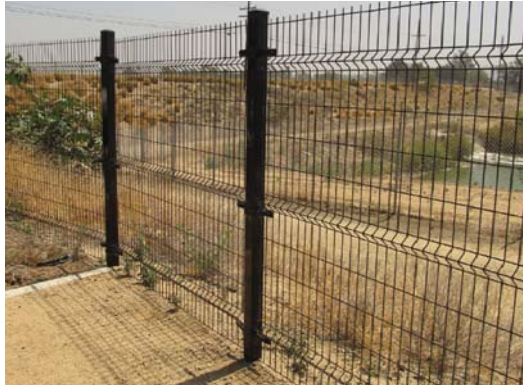
Low-carbon steel wire mesh safety fencing
