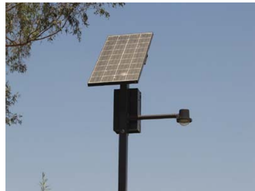
Solar-powered lighting
