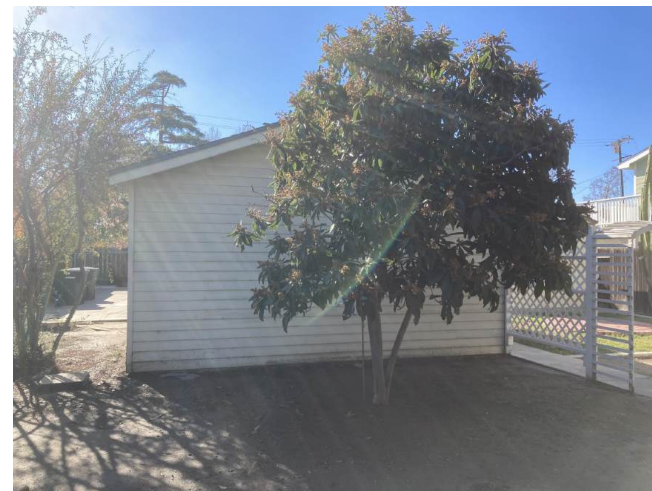
View of north facade of existing garage
