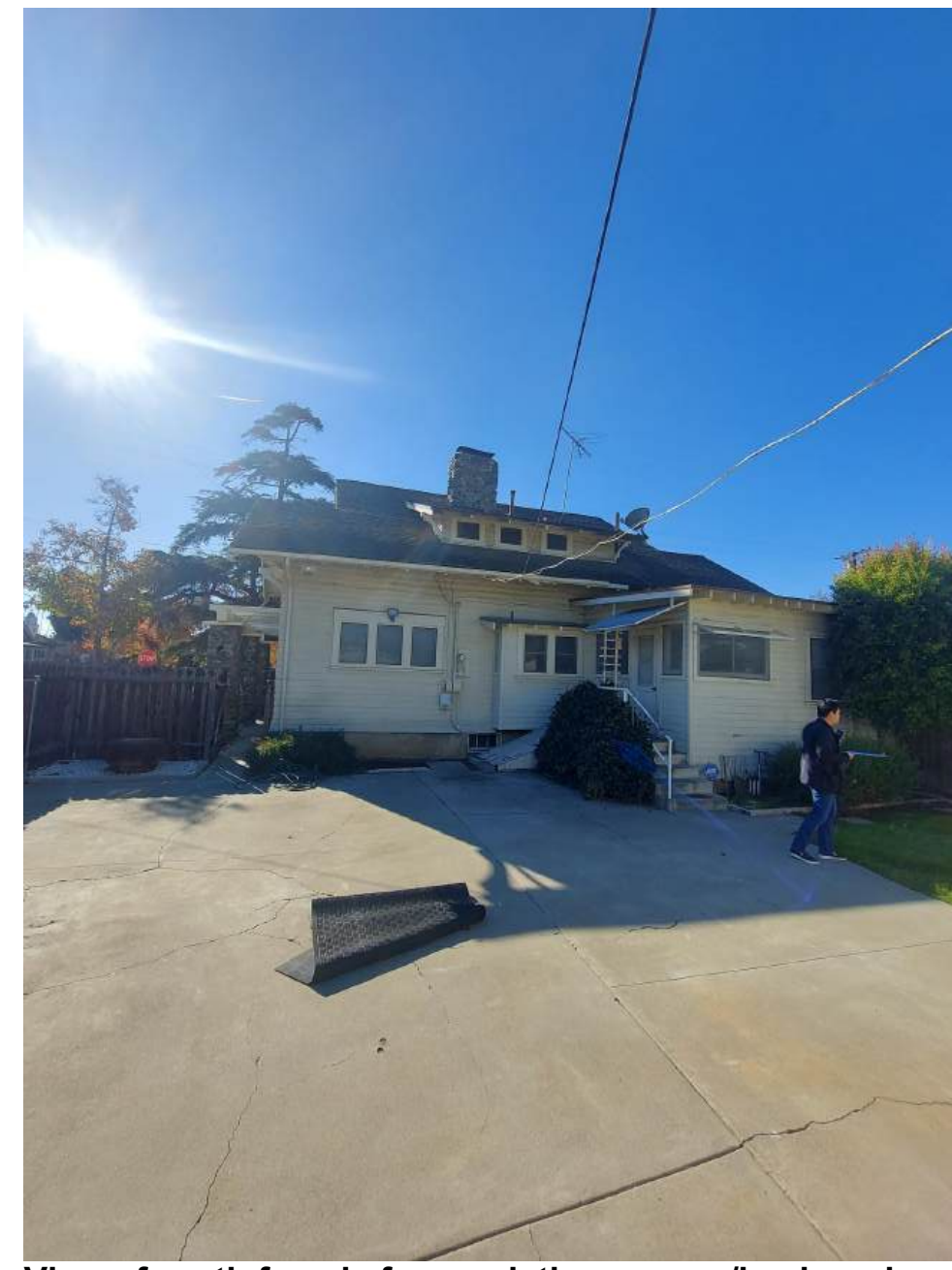
View of north facade from existing garage/backyard
