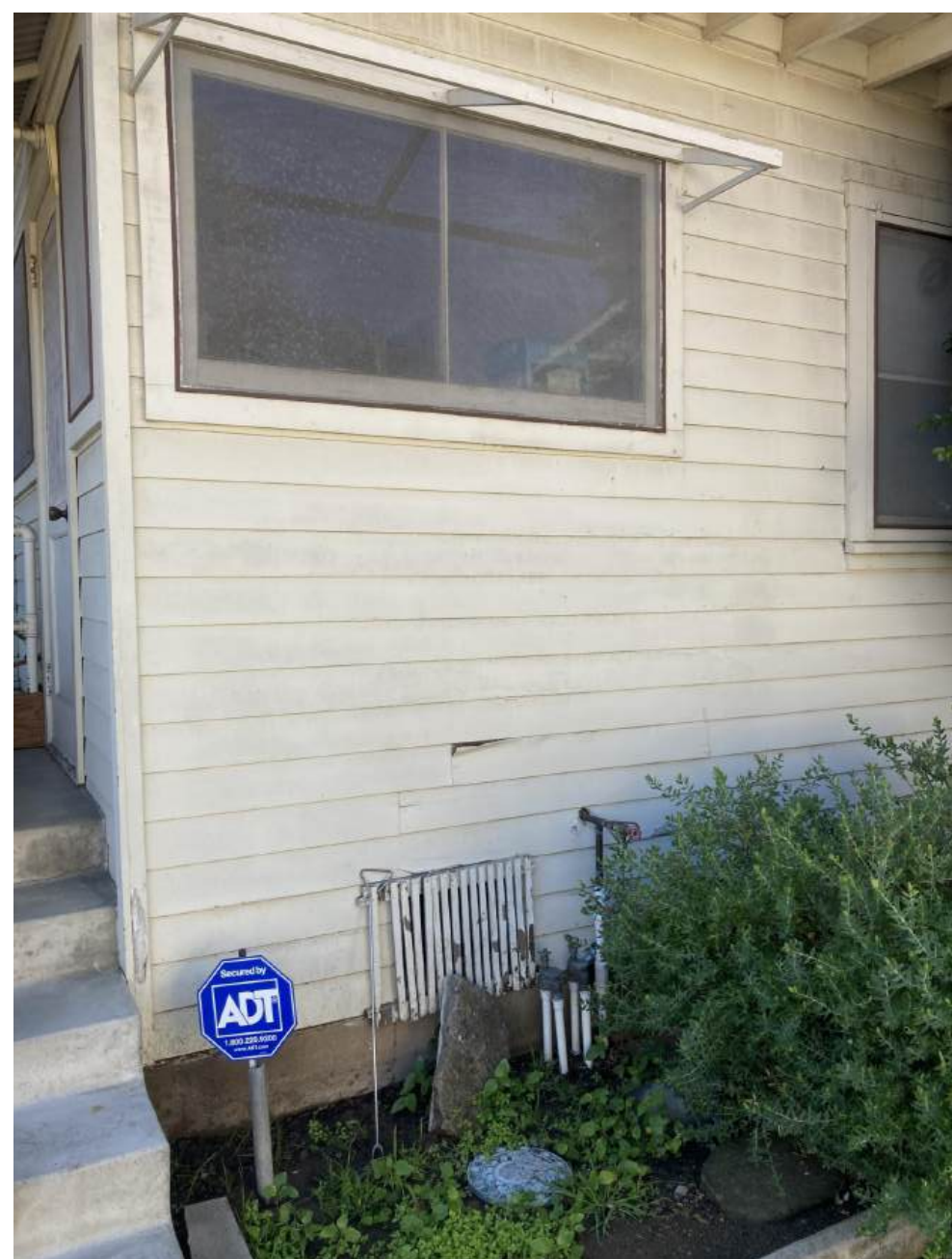
Closeup view of window being replaced at addition
