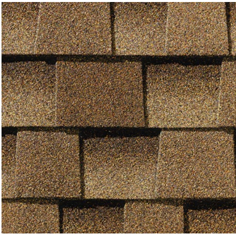
5. Roof Shingles Timberline HD in "Shakewood"
