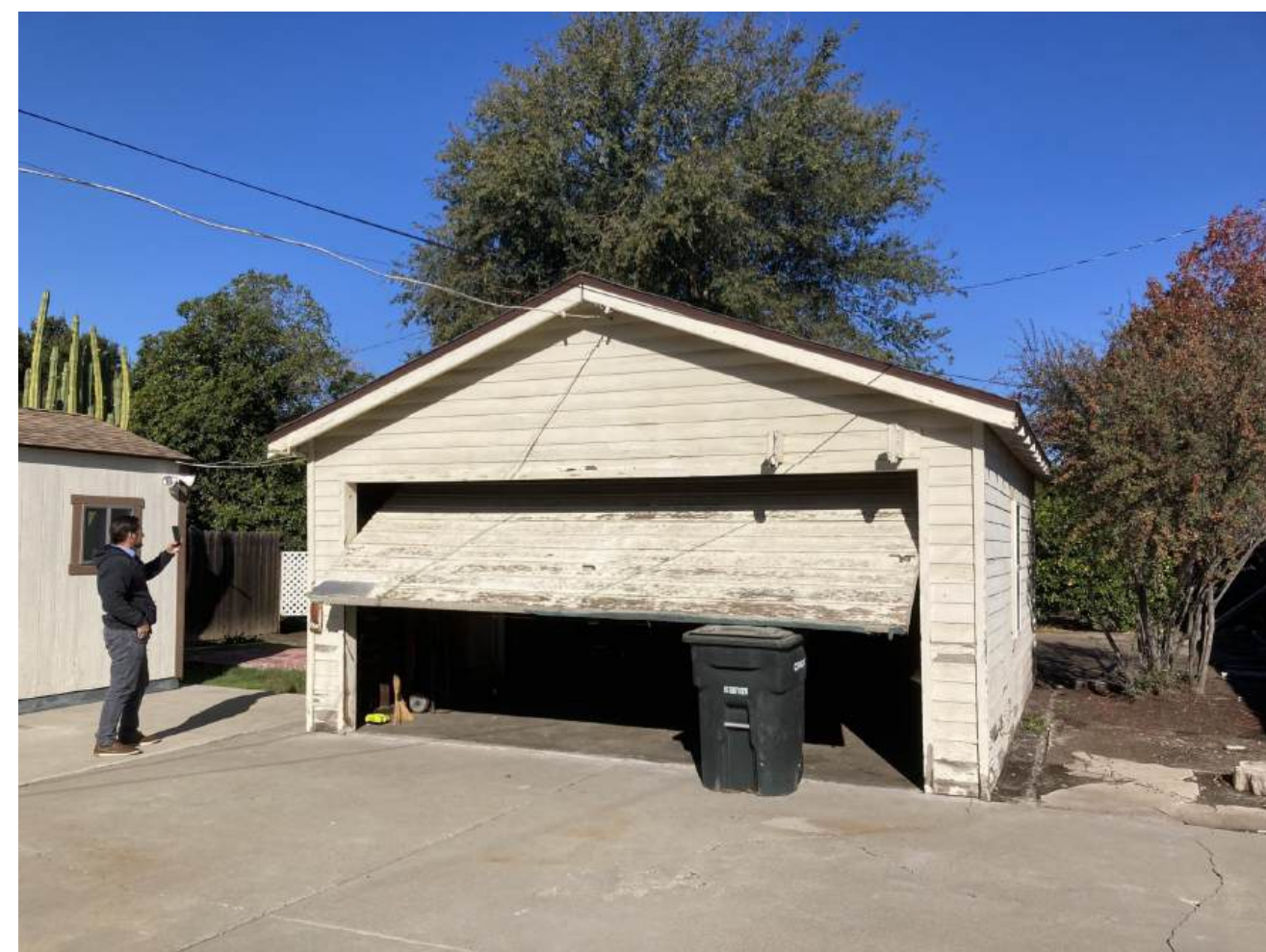
View of south facade of existing garage
