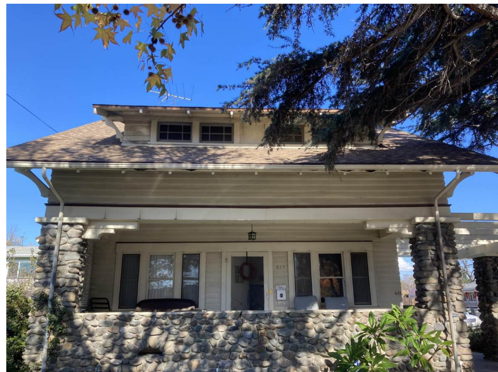
Closeup view of south facade of main residence
