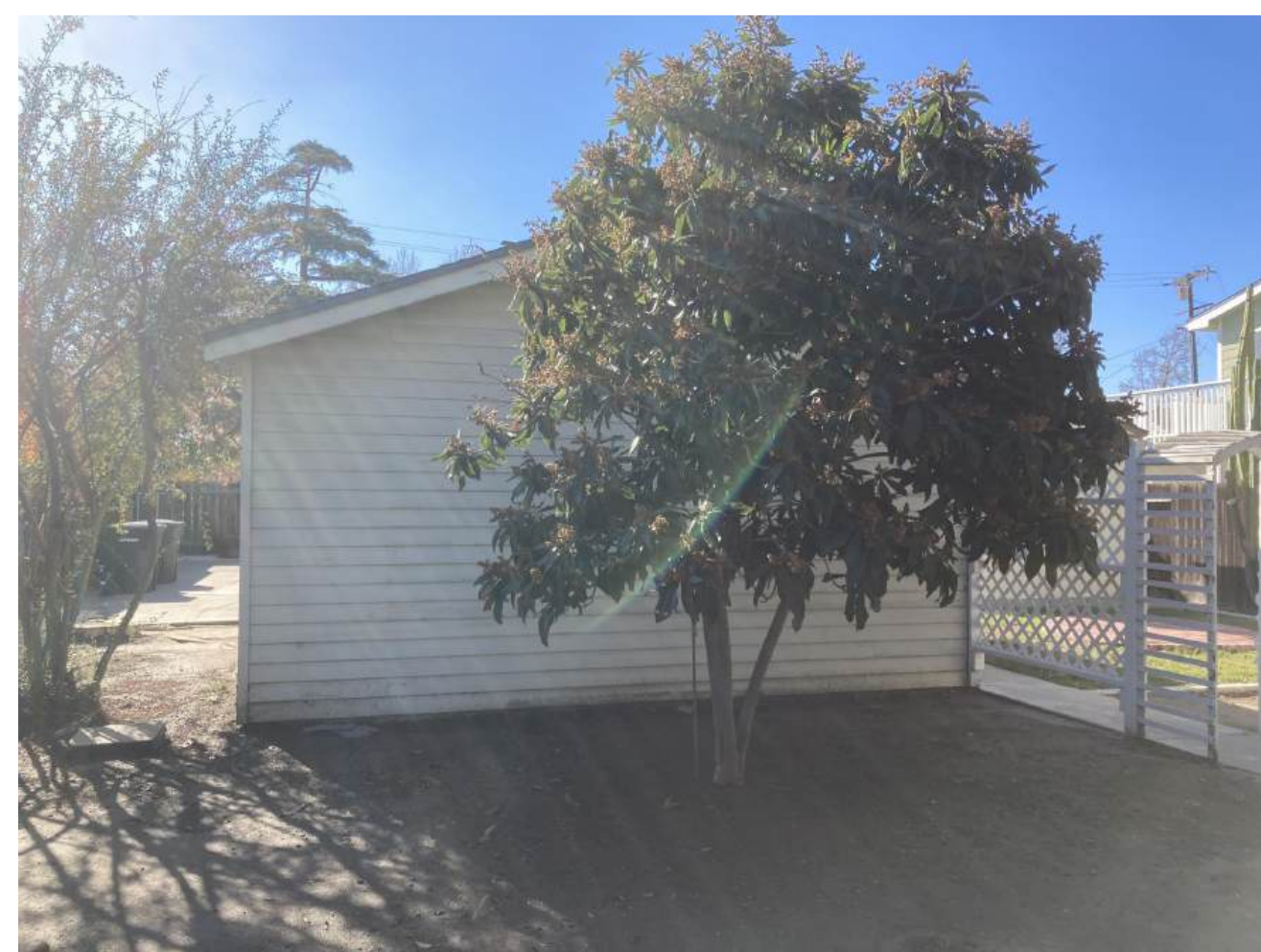
View of north facade of existing garage
