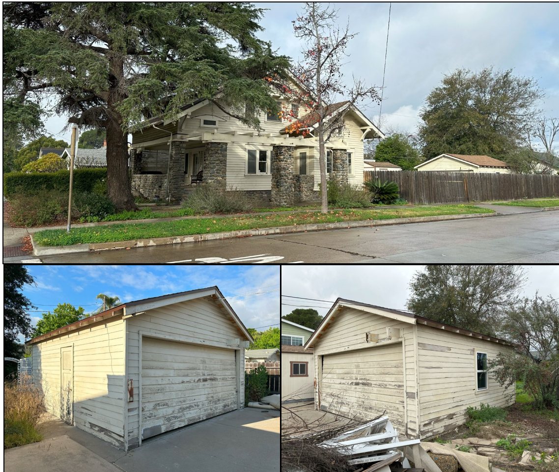
Charles and Alice Parker House Property, Rear Garage
