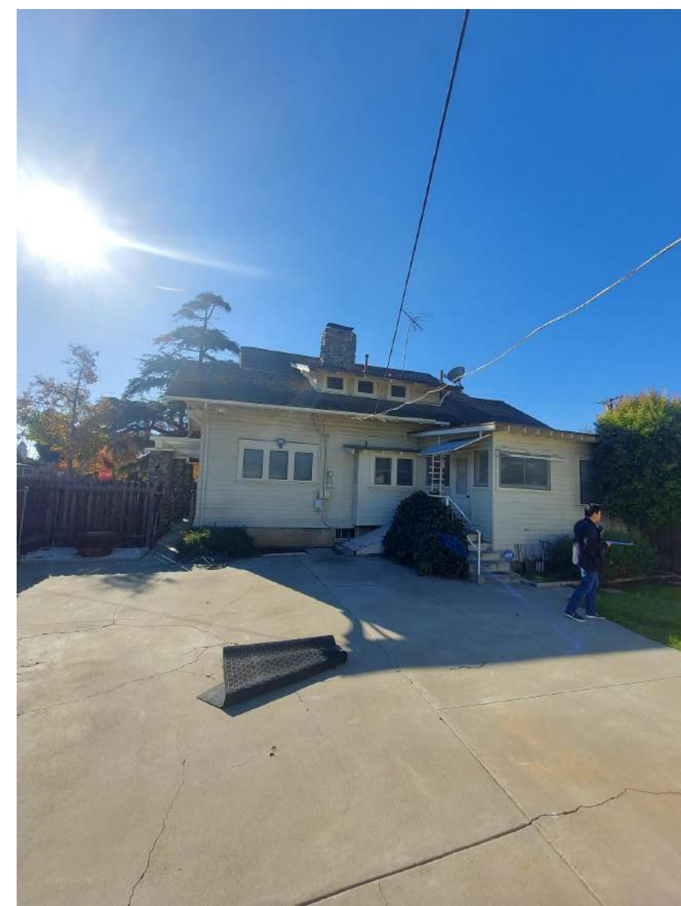
View of north facade from existing garage/backyard
