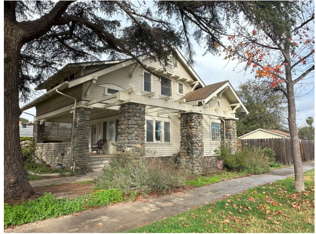
Façade, east elevation, and garage, view northwest
