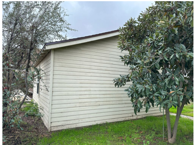
Garage rear elevation, view south/southwest
