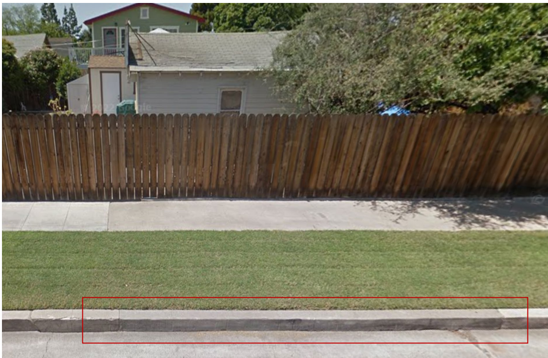
Section of Curb Infill at Previous Driveway
