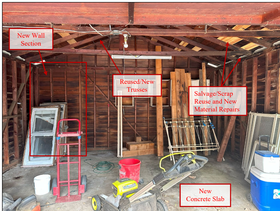
Charles and Alice Parker Garage Interior, Rear Elevation
