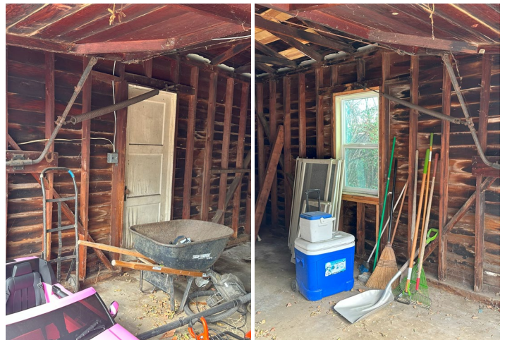
Garage interior west & east elevations, respectively, view NW & NE
