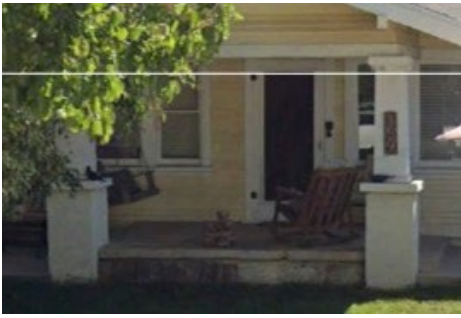
154 N Harwood Stucco masonry pilasters
