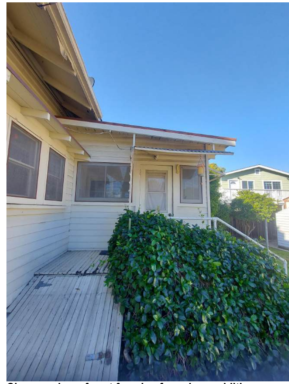
Closeup view of east facade of previous addition
