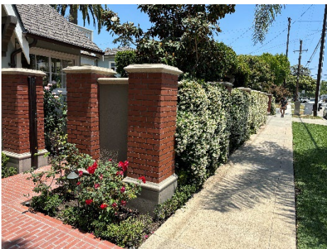
205 Pine St Solid wall with pilasters
