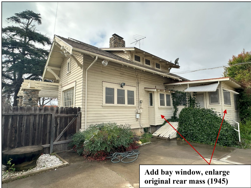
Charles and Alice Parker House Rear Modifications
