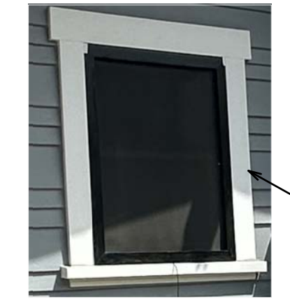
WOOD DOUBLE HUNG, DUAL GLAZED COLOR: DEN 340, WHITE WITH DARK WOOD SCREENS (WALNUT STAIN)
