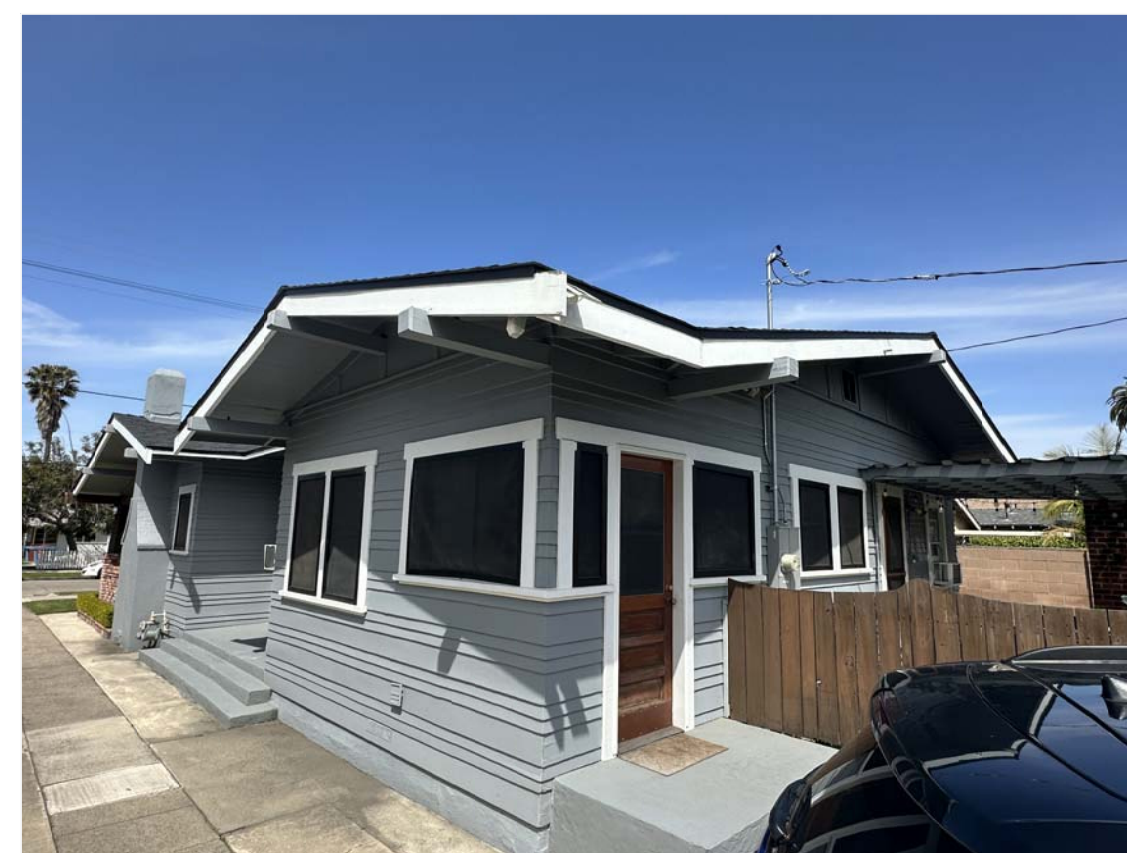
4 VIEW LOOKING NORTH WEST
