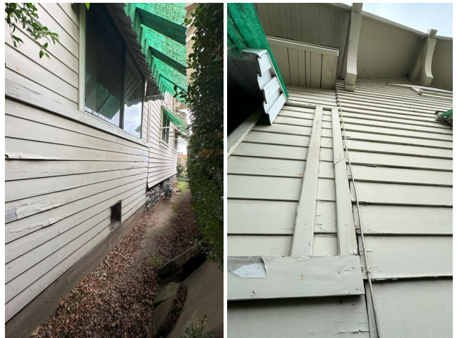
West elevation, showing addition/modificaton & detail, view S & SE
