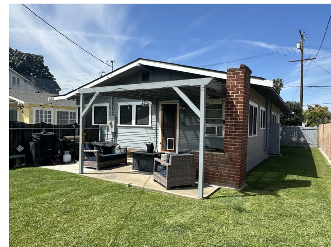
8 VIEW LOOKING SOUTH-WEST
