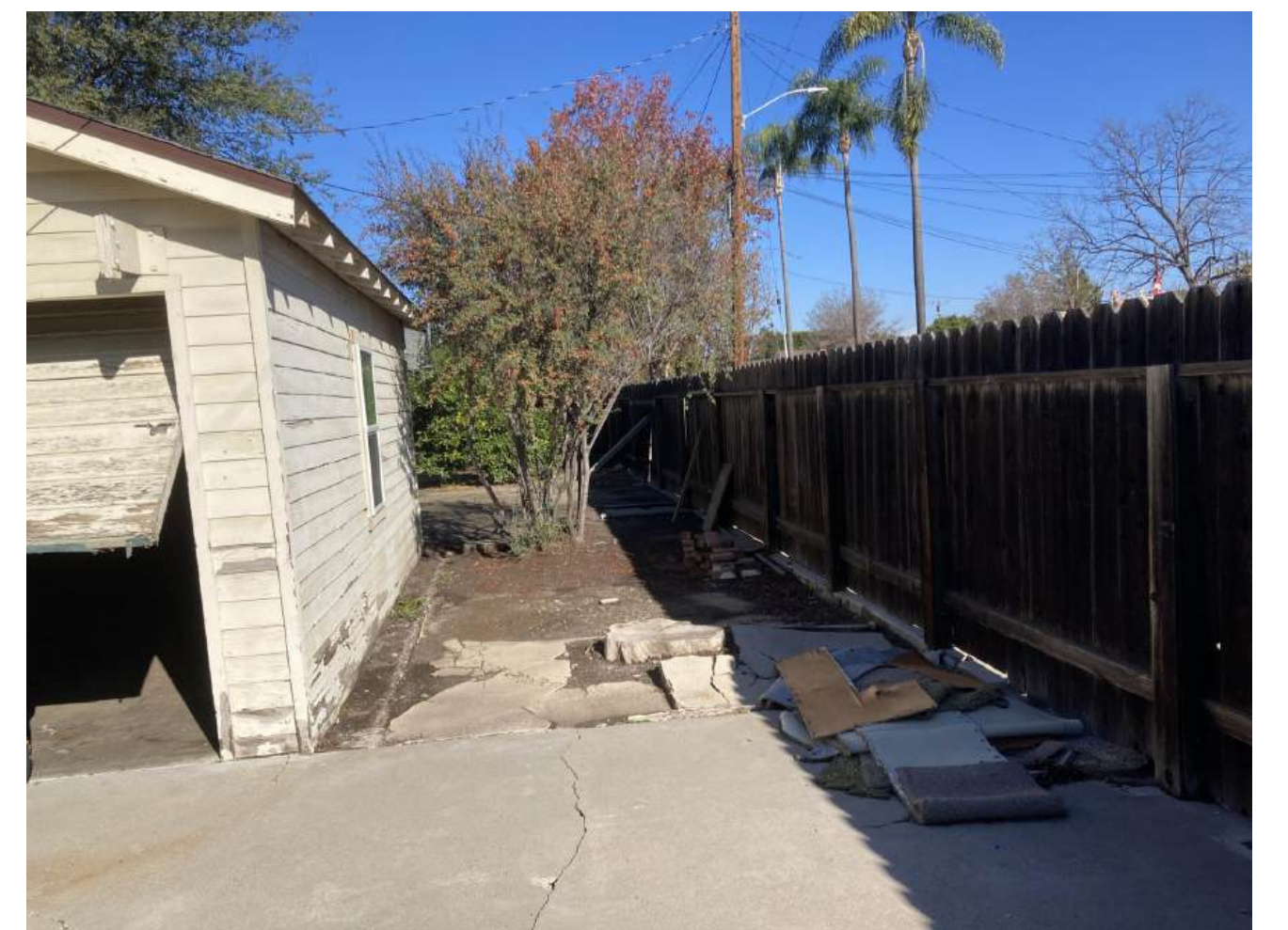
View of east facade of existing garage
