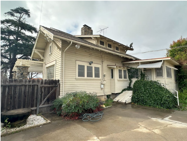
Rear elevation, showing additions/modifications, view southwest
