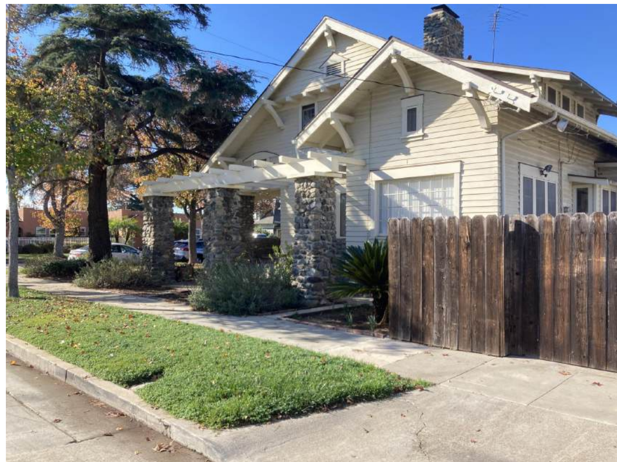
View of east facade from street
