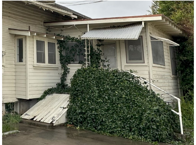
Rear elevation modifications detail, view west/southwest
