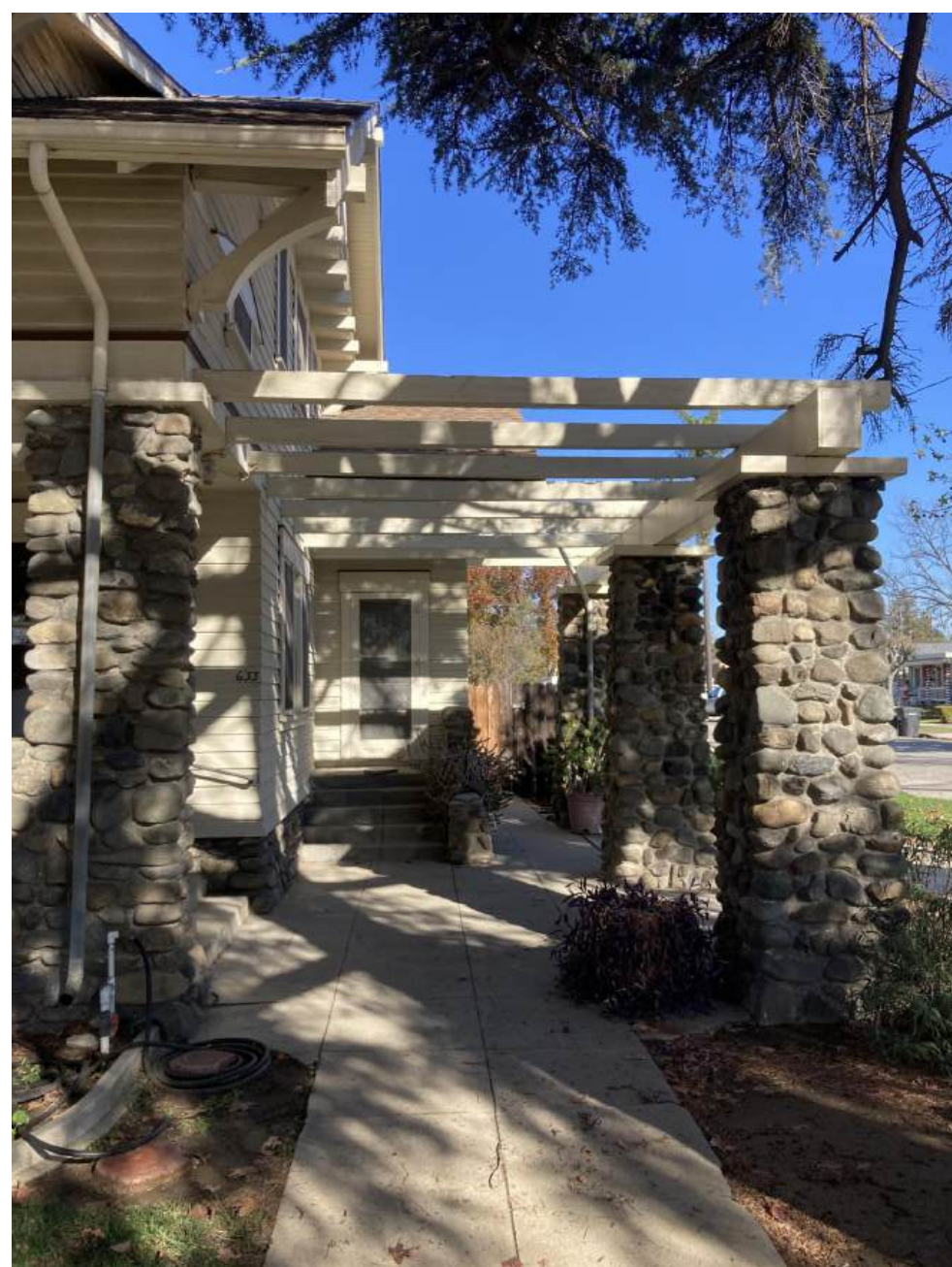
View of trellis at southeast corner of residence being restored
