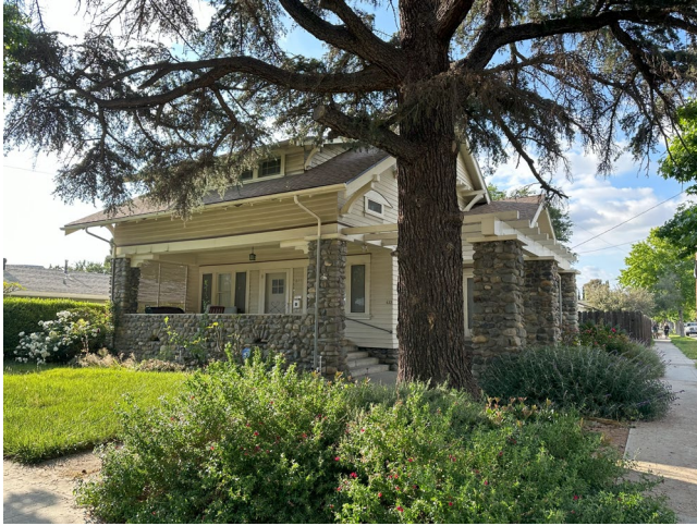
Façade & east elevation, view north/northwest
