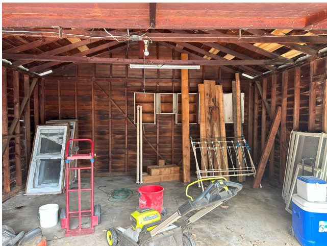
Garage interior rear elevation, view north
