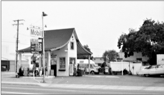
Figure 8: 305 S. Main with sheds (far right). Source: Orange County Archives.
