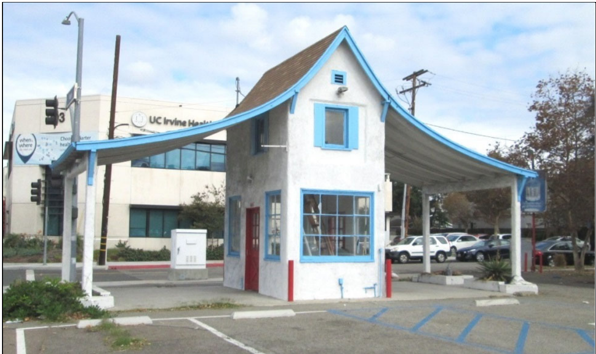
Figure 11: Former gas station, south and west elevations, view to the northeast (10/31/17).
