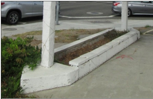
Figure 15: West pump island, view to the northwest (10/31/17).
