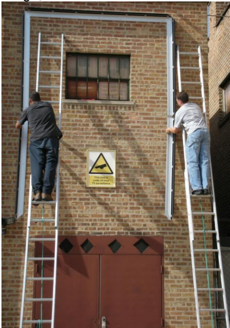
Mounting frame sides to our building.
