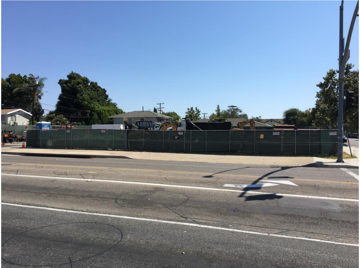
North property line facing south, across E. Collins Avenue.
