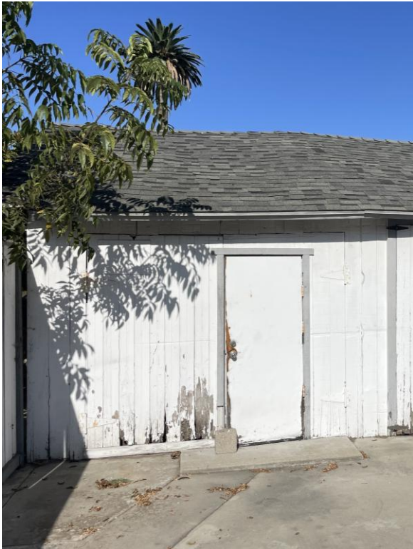
Figure 7. Detail view of primary (east) façade of garage with flush vertical boards as the siding around the garage opening, view west.
