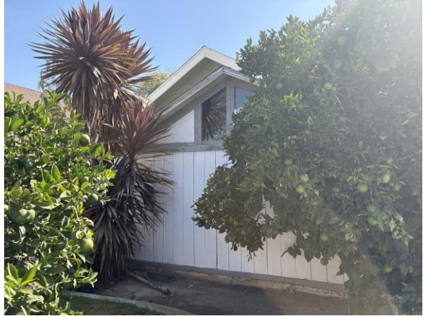
Figure 15. West façade of ancillary building, view northeast.
