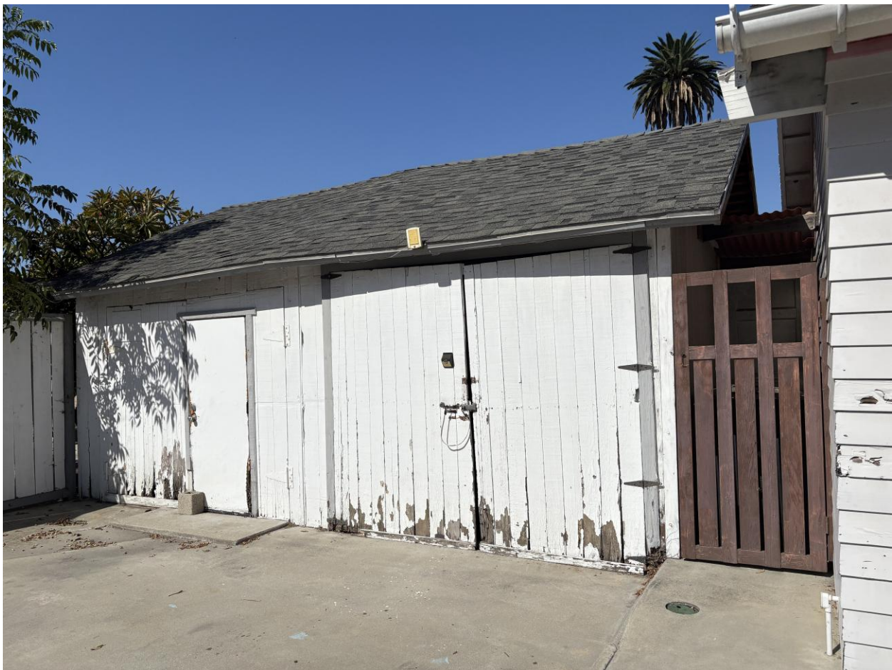
Figure 6. East façade of the garage, view southwest.
