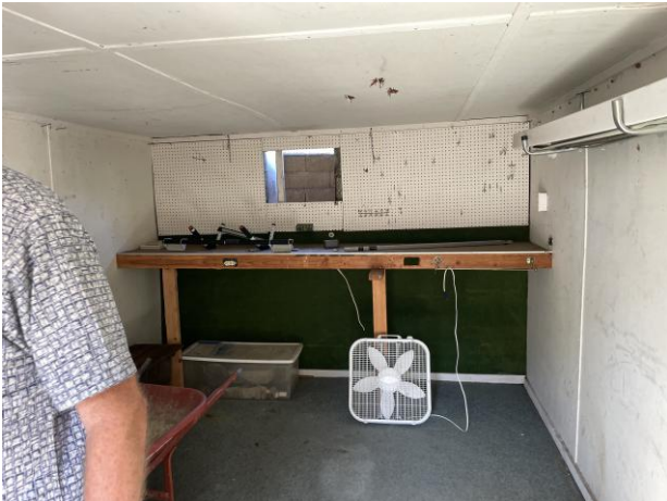
Figure 11. Interior of the south garage bay, view west.
