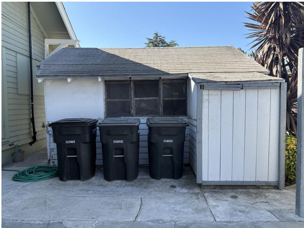
Figure 13. North façade of ancillary building, view south.
