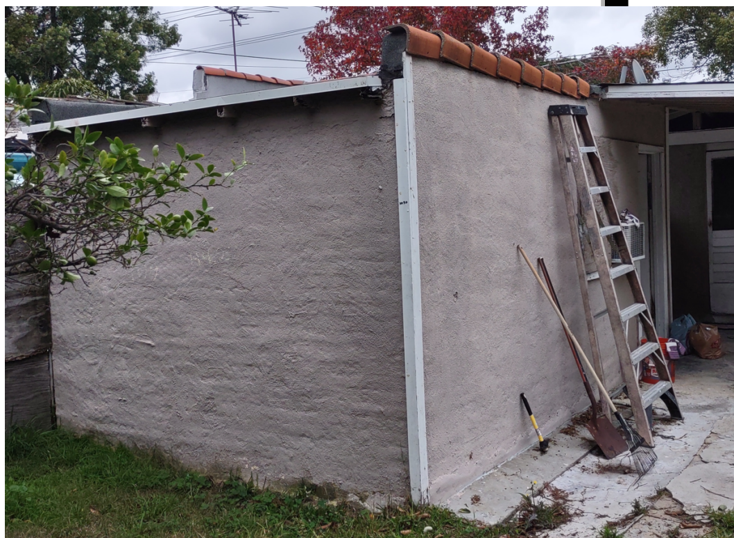
GARAGE REAR AND SIDE FROM THE WEST
