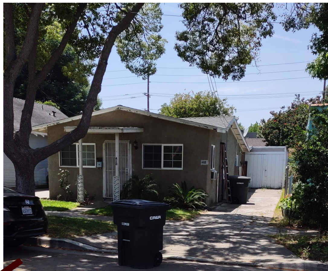
FRONT AND SIDE / GARAGE FROM NORTHEAST
