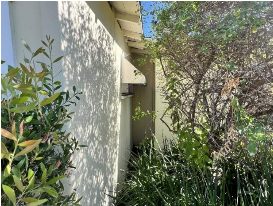
Figure 13: West façade of 173 North Waverly Street [facing south]. Source: JANUS
