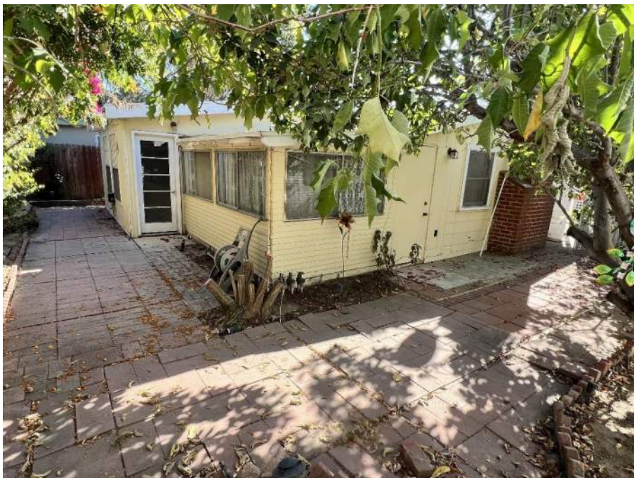
Figure 08: Northeast corner of 173 North Waverly Street [facing southwest]. Source: JANUS
