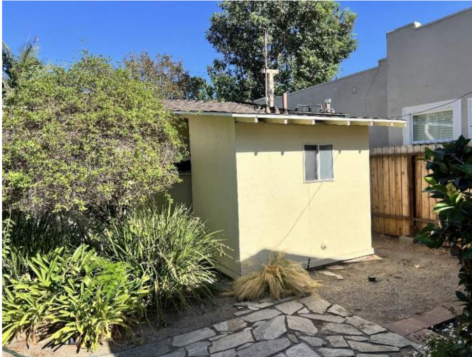
Figure 12: West façade of 173 North Waverly Street [facing southeast]. Source: JANUS
