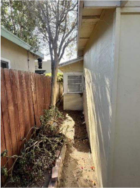
Figure 09: South façade of 173 North Waverly Street [facing west]. Source: JANUS
