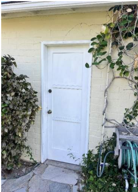
Figure 16: Existing door at north garage façade [facing south]. Source: JANUS
