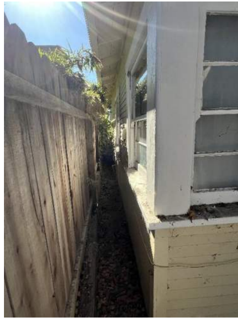
Figure 10: South façade of 173 North Waverly Street [facing west]. Source: JANUS
