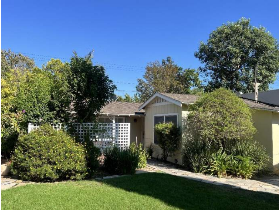
Figure 05: 173 North Waverly Street [facing southeast]. Source: JANUS
