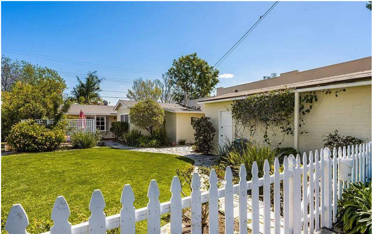
Figure 01: Street view of 173 North Waverly Street [facing east-southeast].
