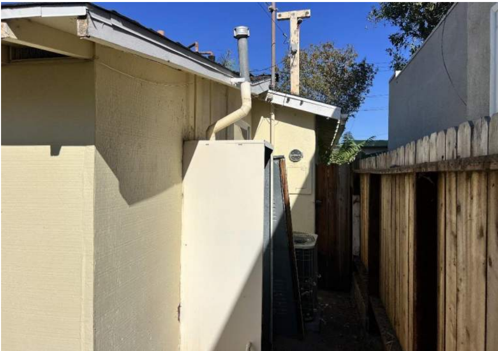
Figure 11: South façade of 173 North Waverly Street [facing east]. Source: JANUS
