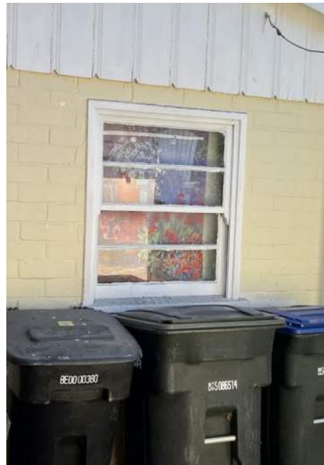
Figure 17: Existing window at east garage façade [facing west]. Source: JANUS
