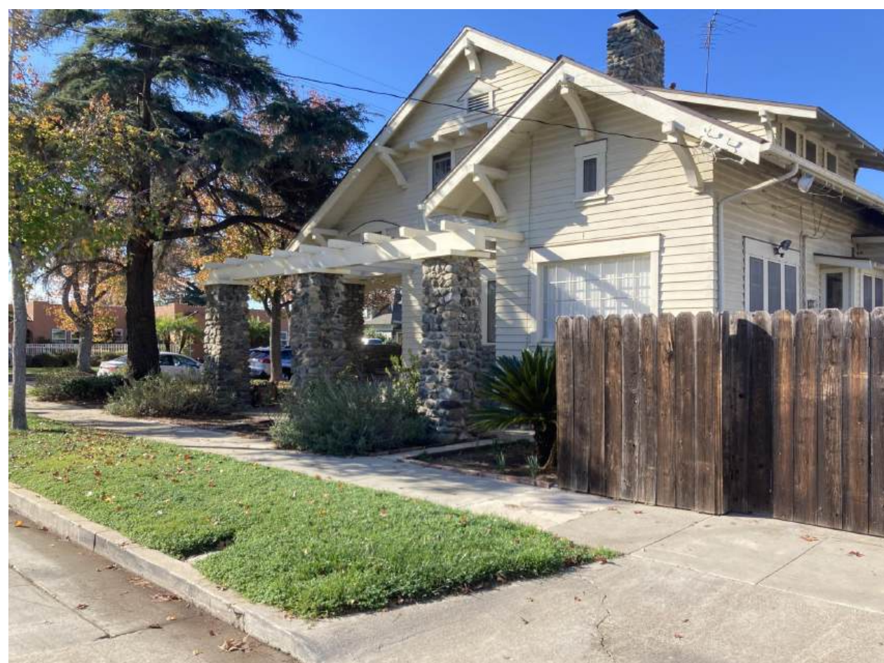
View of east facade from street
