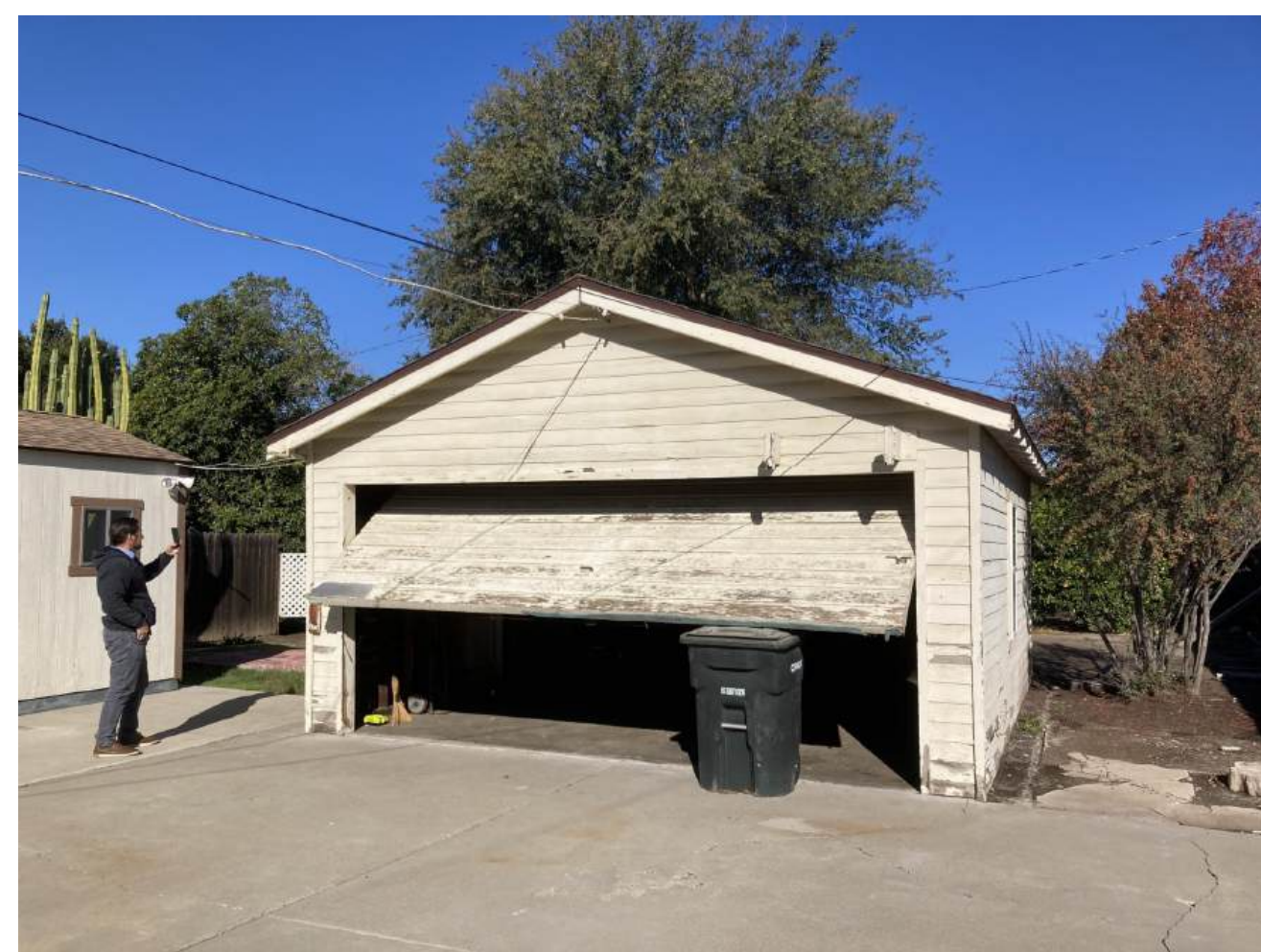
View of south facade of existing garage
