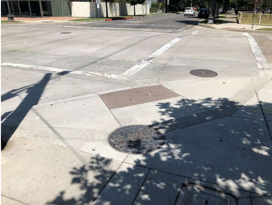
The City may want to change out this manhole cover for one without the raised pattern for better ADA compliance
