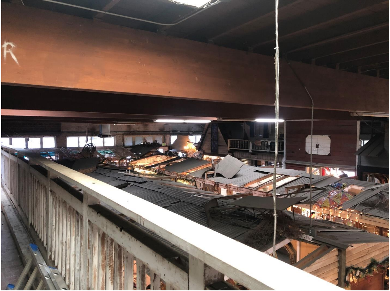
12. View from interior mezzanine / Open rafter ceiling and wood glulam beams, 204 W. Chapman Avenue (view northeast); December 14, 2020
