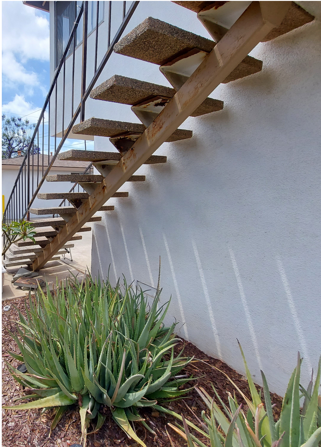
View of Deteriorated Staircase
