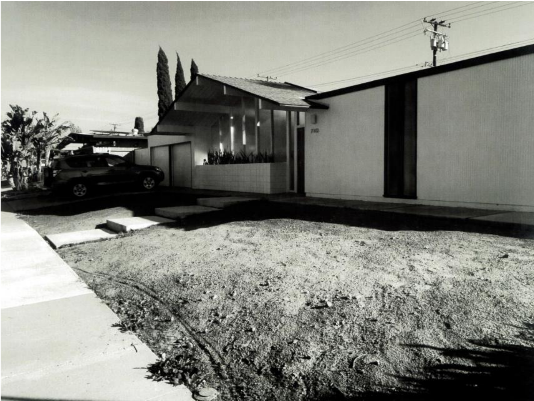
MAC-388.0-21 - 710 E. Palmdale Avenue
