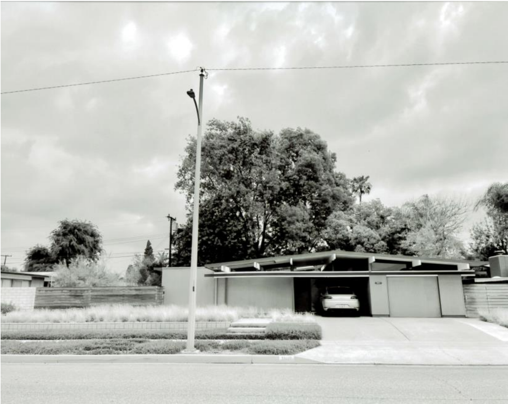
MAC-390.0-21 - 1801 N. Woodside Street
