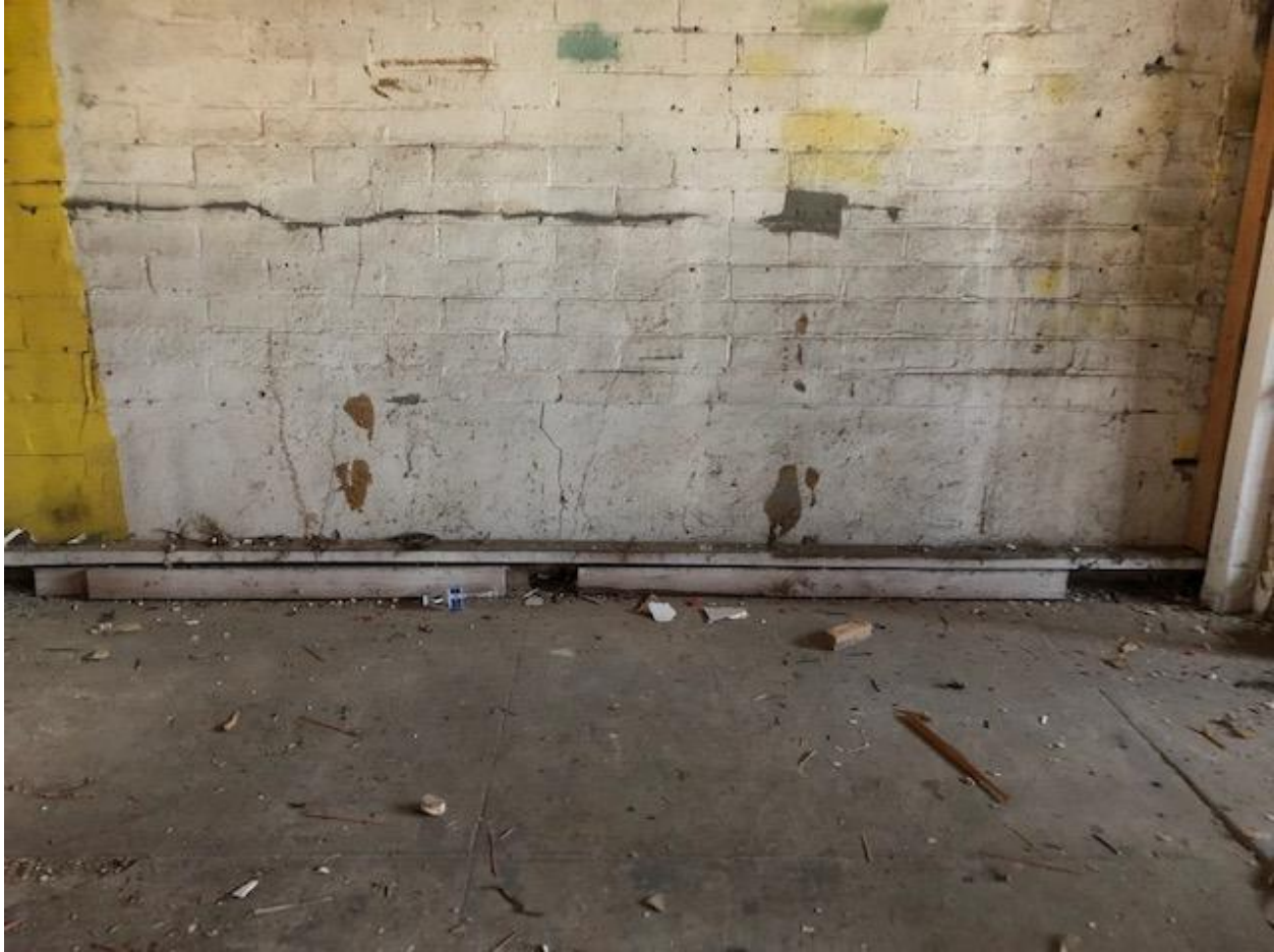
Figure 4C. Window Infill/Building Scarring (interior view)
