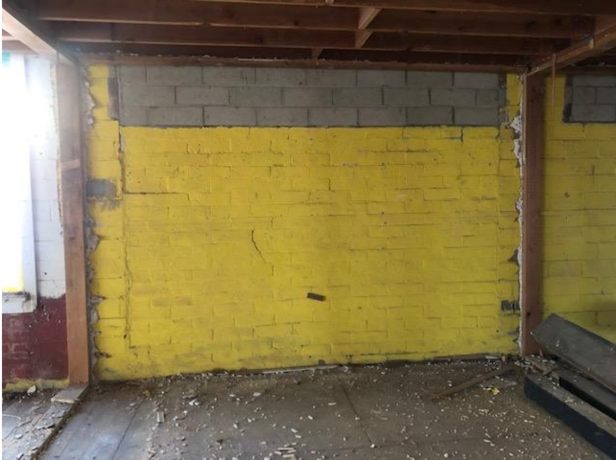
Figure 4A. Window Infill/Building Scarring (interior view) SOURCE: Sapphos Environmental, Inc., 2021
