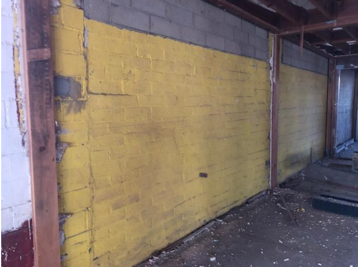
Figure 4B. Window Infill/Building Scarring (interior view) SOURCE: Sapphos Environmental, Inc., 2021
