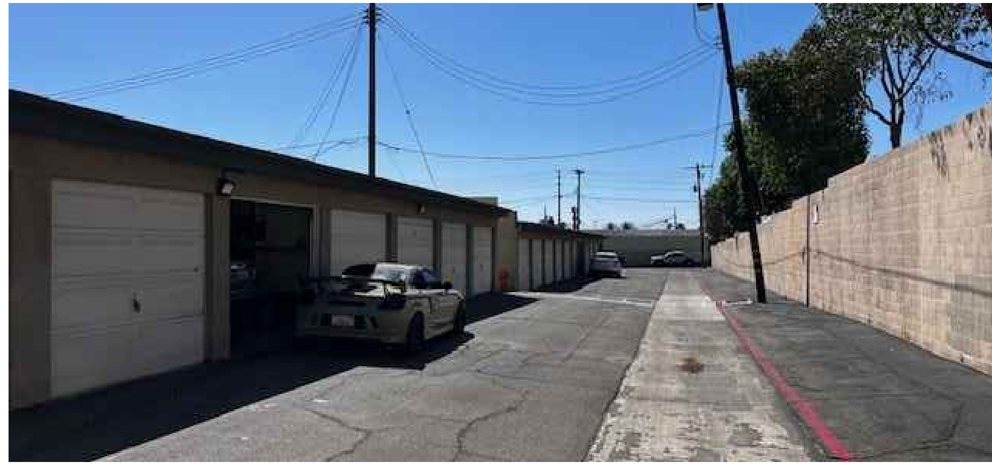
IEWS OF ADJACENT GARAGES SOUTH OF LOT 9
