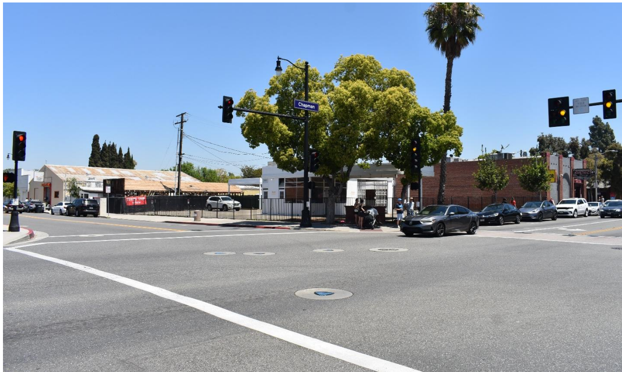
Image 1: Project Site, view northeast from West Chapman Avenue and North Lemon Street
