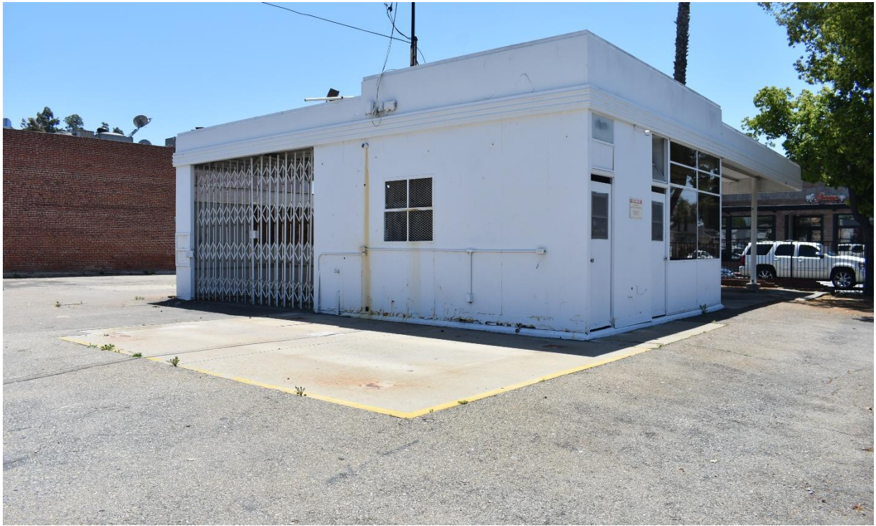
Image 4: Building B, north and west façades, view southeast
