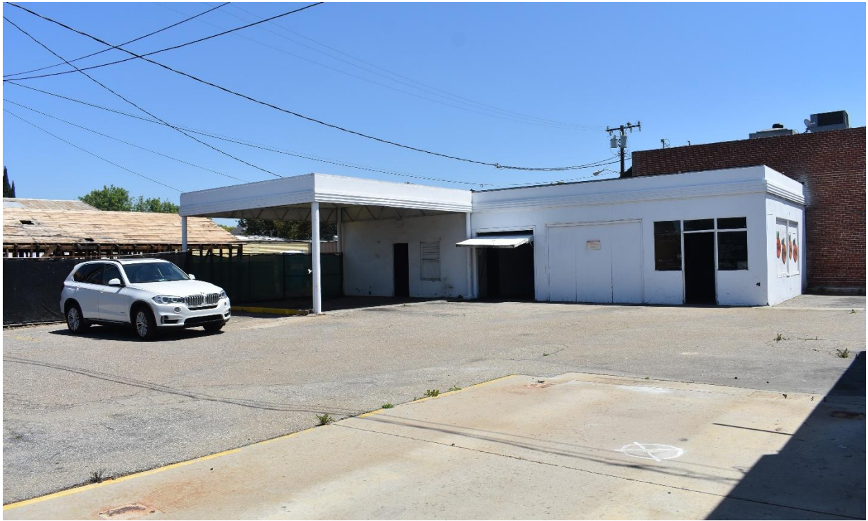
Image 2: Building A, south and west façades, view northeast
