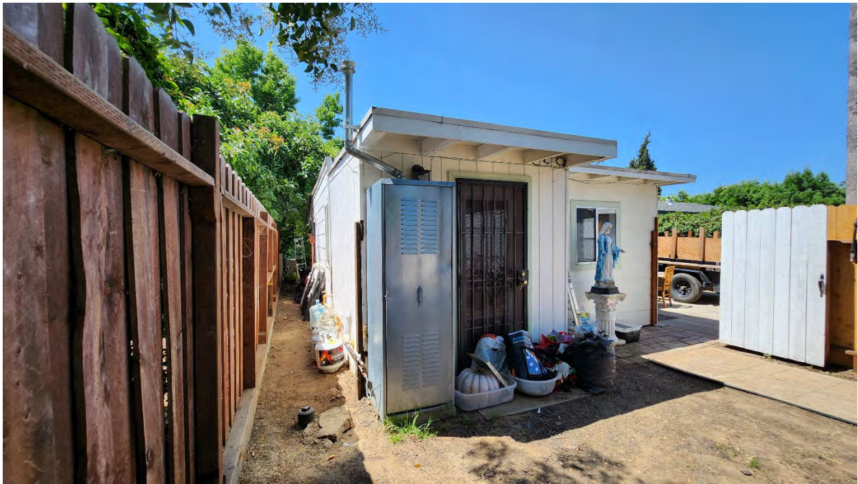
Figure 8: East (left) and north (right) elevations, view facing southwest. Source: GPA Consulting, July 2024.
