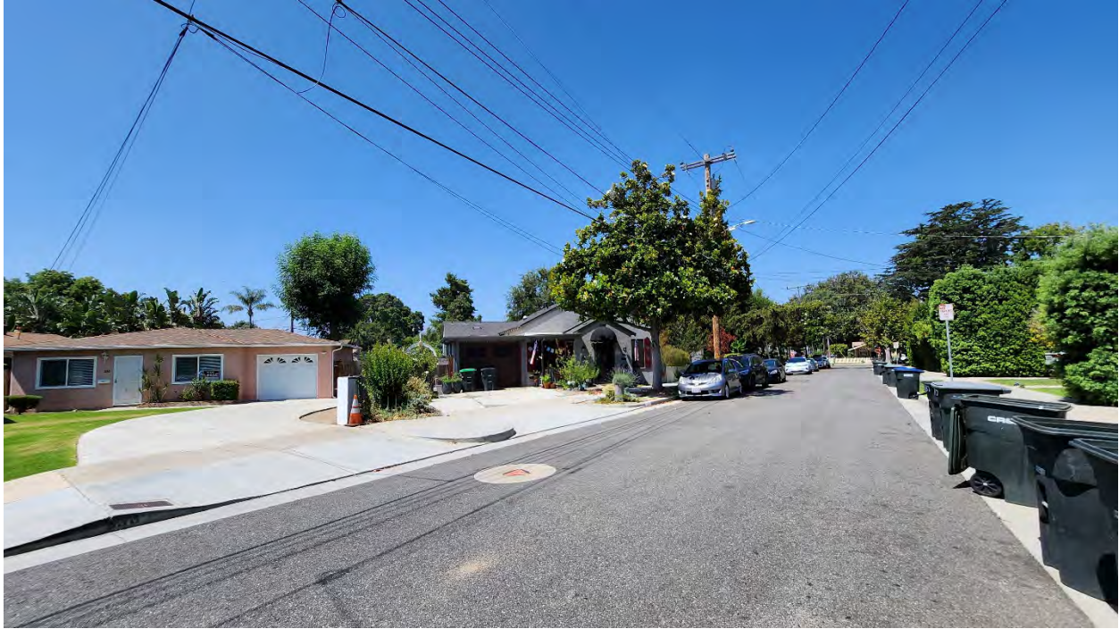
Figure 3: E. Toluca Avenue, view facing southwest from subject property toward nearby contributor, 334 E. Toluca Avenue. Source: GPA Consulting, July 2024.
