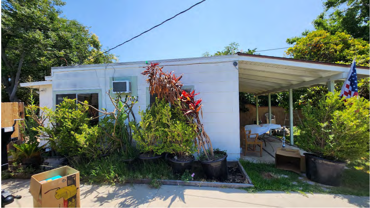
Figure 11: West elevation, view facing east. Source: GPA Consulting, July 2024.
