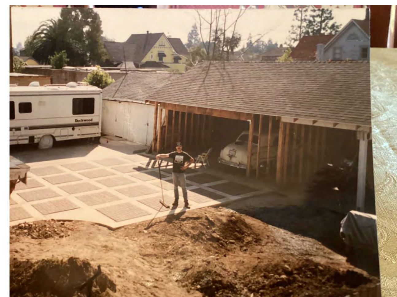
CONSTRUCTION PHOTO OF ADJACENT NEIGHBOR GARAGE
