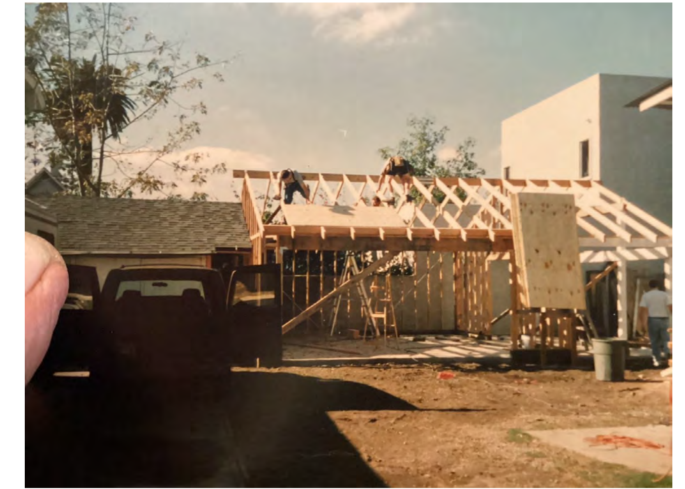
FRAMING OF ADJACENT NEIGHBOR GARAGE
